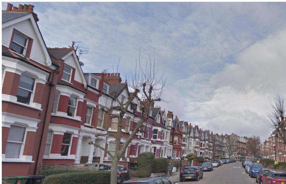
View along west side of Lyncroft Gardens, showing roof slopes concealed by gables and dormers
