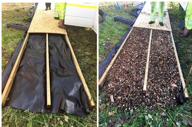
Figure 3. Plywood sheeting used as ground protection.
