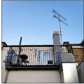
existing balustrade on no.123
