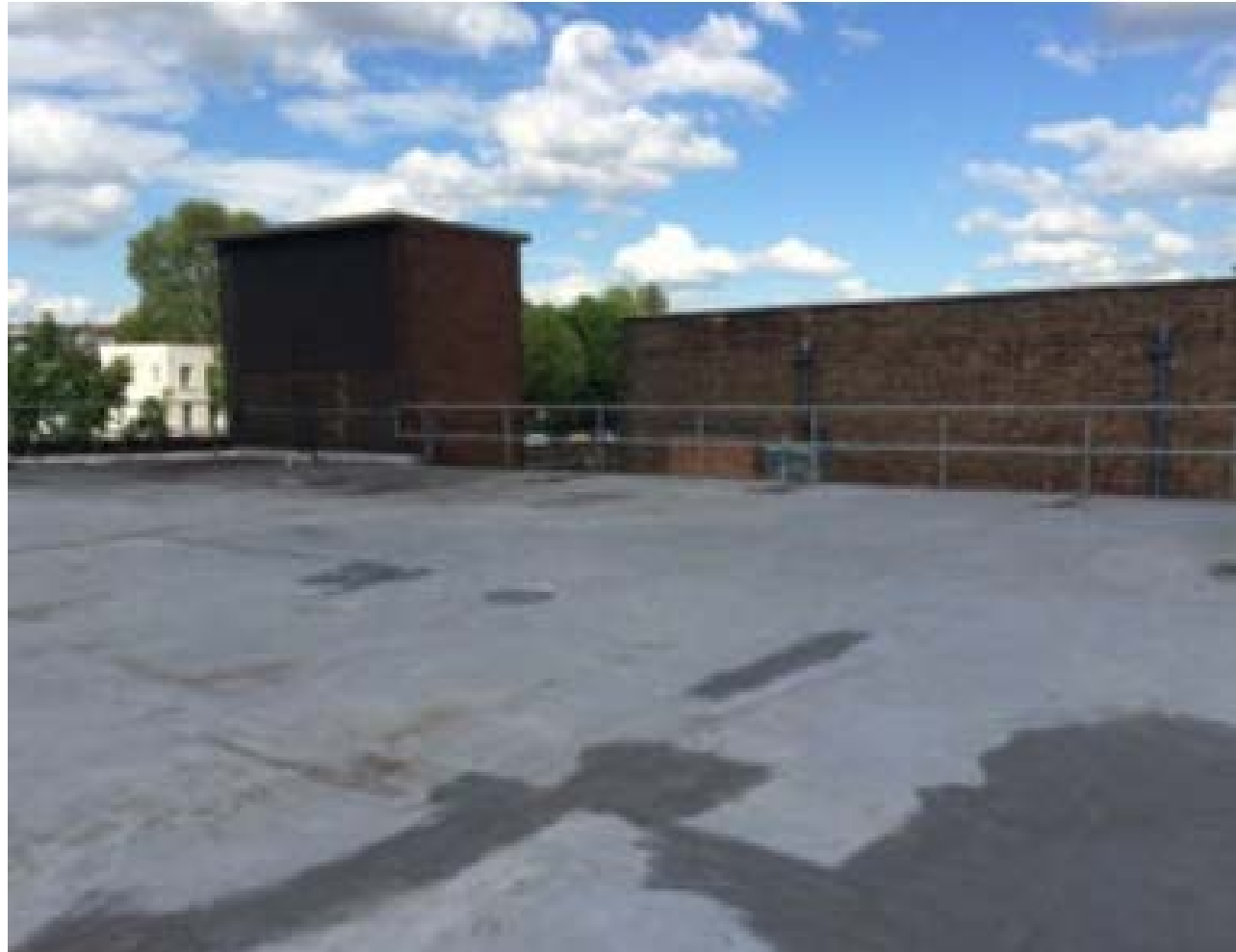
Above: The existing roof above the station.
