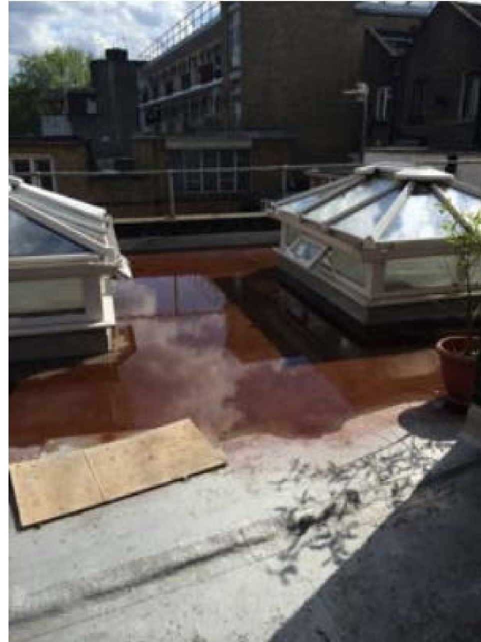
Above: The existing rooflights that would be replaced
