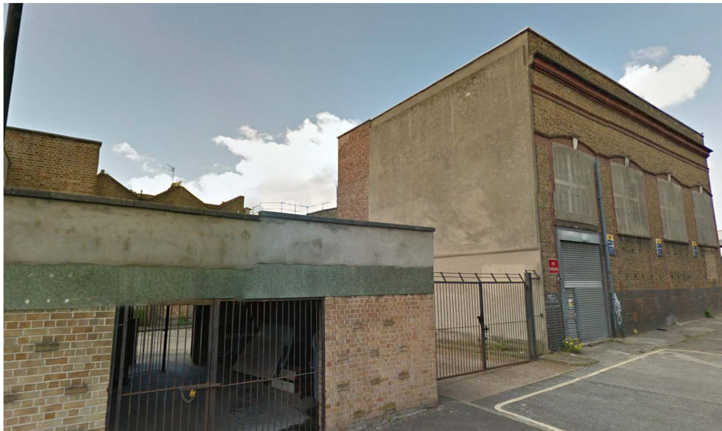
Above: The rear elevation of the Kentish Town Underground Station is obscured from Frideswide Place by a two storey building to the rear.
