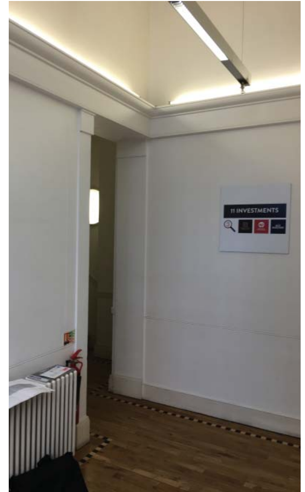
2.4 Access to staircase
