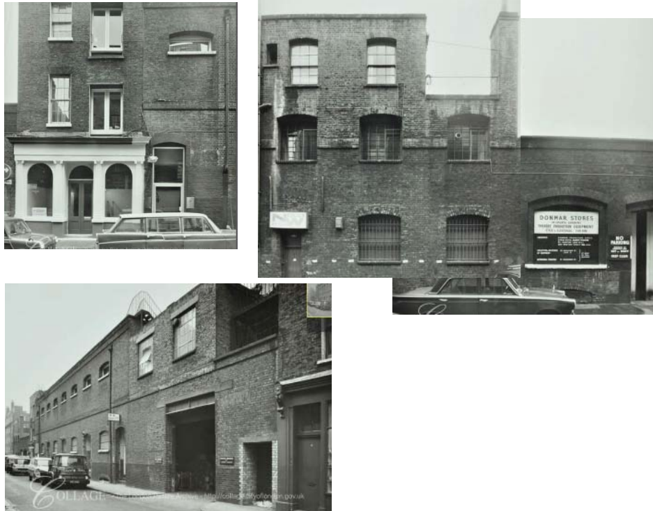
Historic photos of nos 16 and 20 Short's Gardens prior to extensions and alterations in the 1990s
