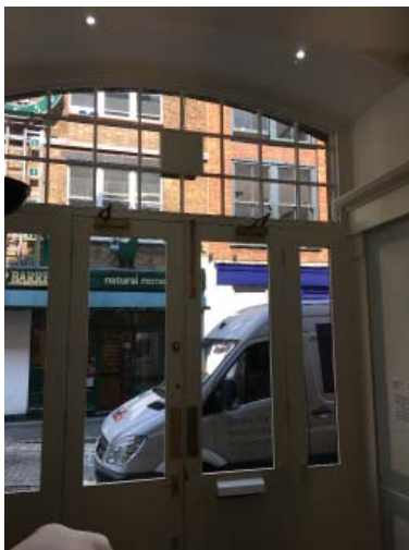
8.1 Entrance and Glazed Door
