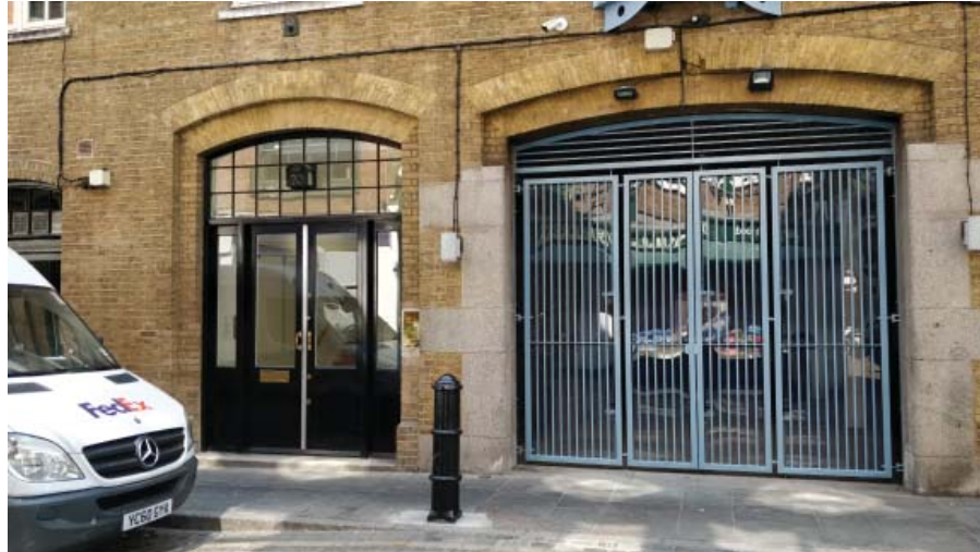
1.2 Entrance outside no.20
