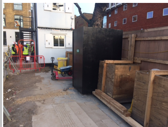
Robust hoarding and temporary concrete ground protection
