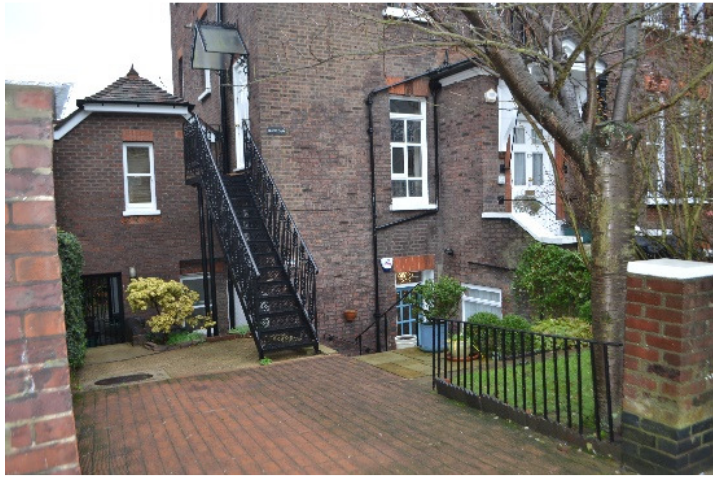
No 12 Daleham Gardens from the street with steps up to 1 st floor flat
