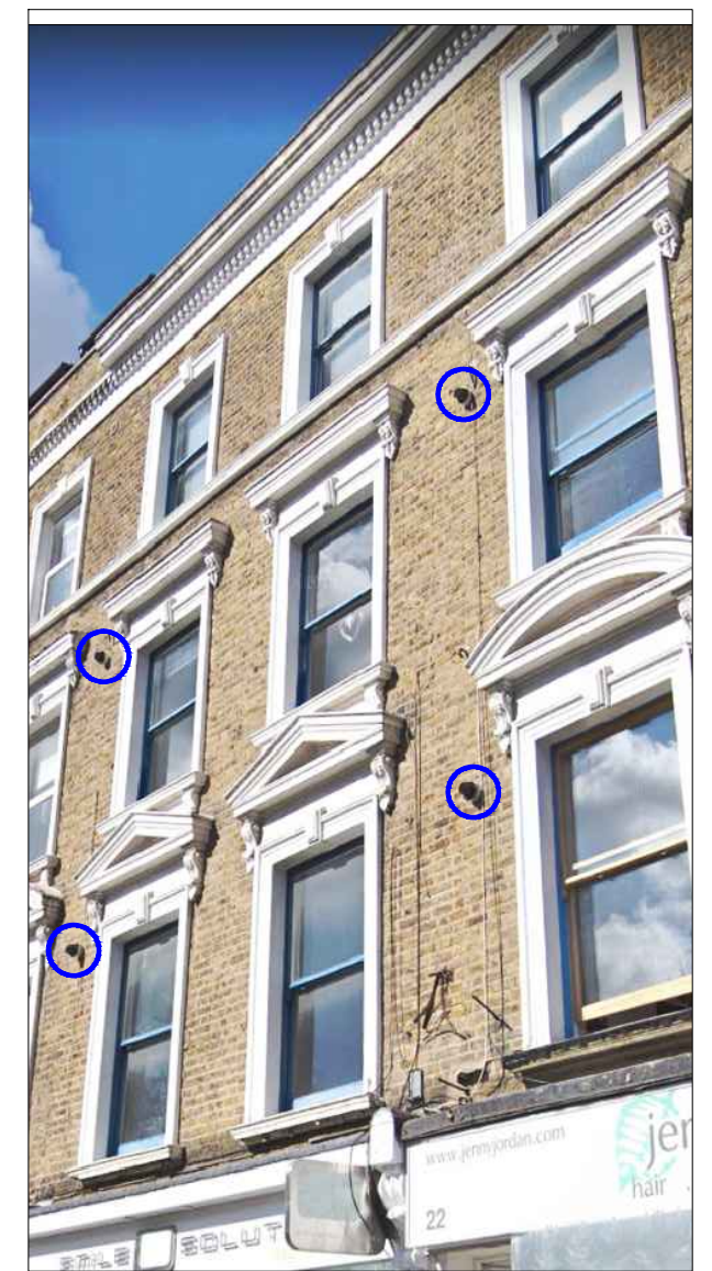
4. FRONT FLUE TERMINALS AT 22 & 24 ENGLAND'S LANE.
