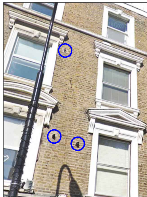
5. FRONT FLUE TERMINALS AT 4 & 6 ENGLAND'S LANE.
