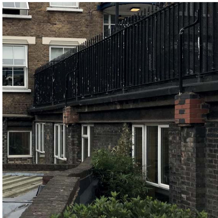
6.4.1 Existing condition - north elevation
