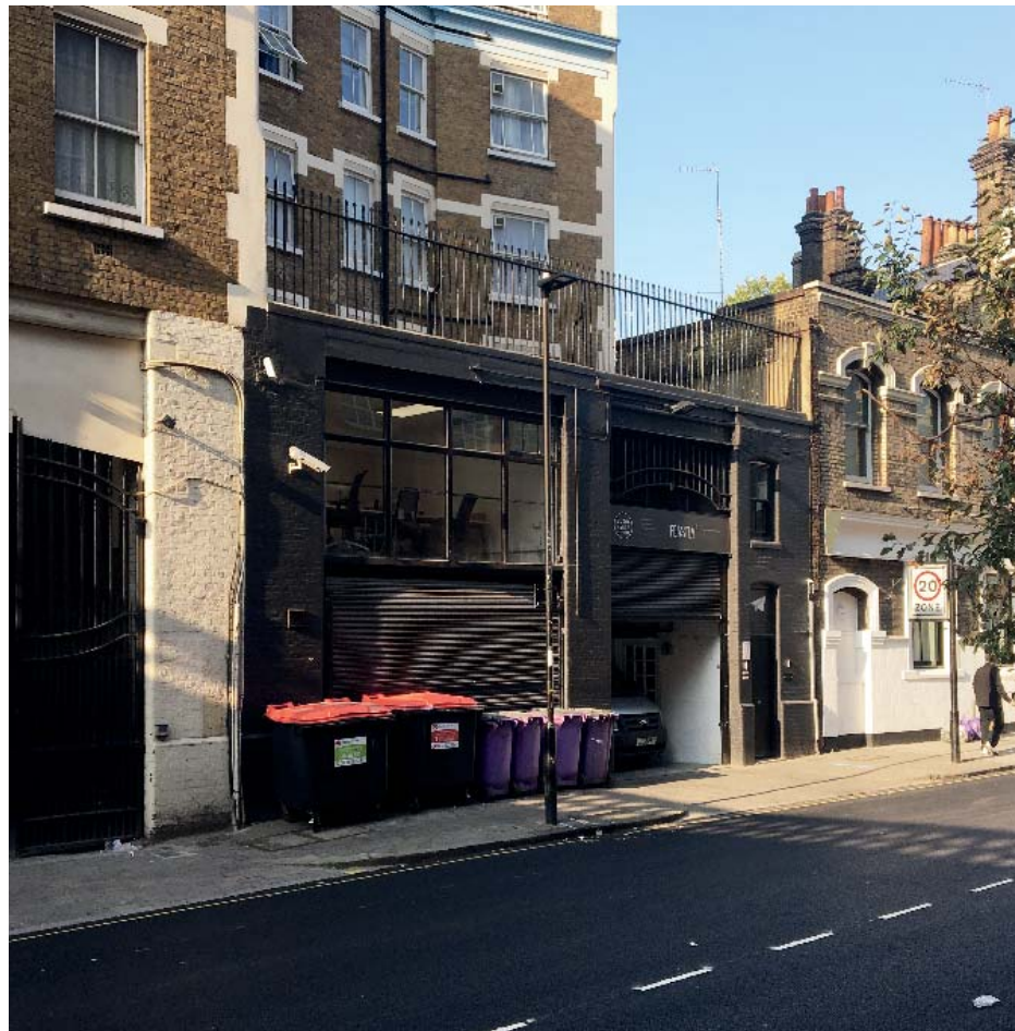
6.2.1 Existing Warner Street facade
