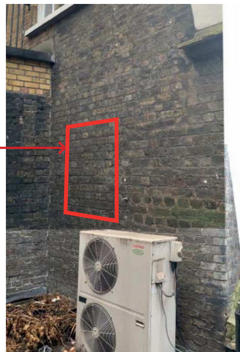
7.1.1 West courtyard view
