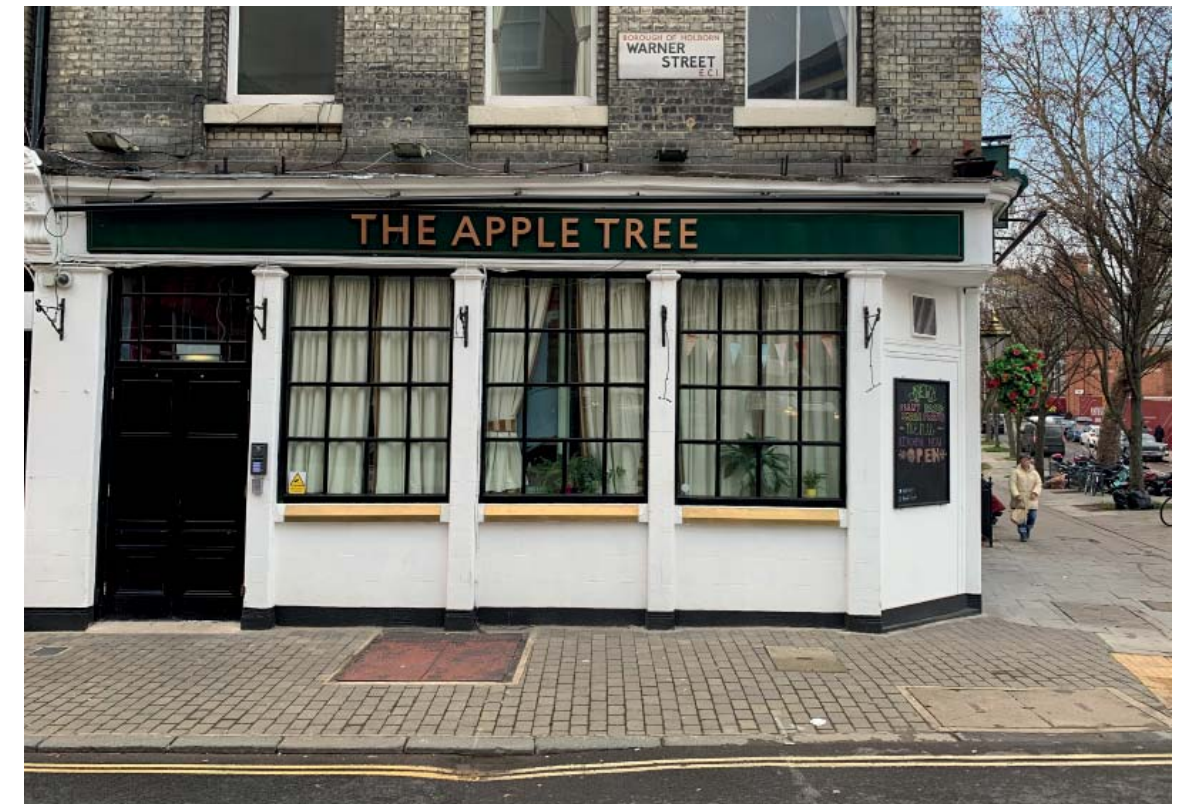
5.1.3 Window grid to ground level The Apple Tree Public House
