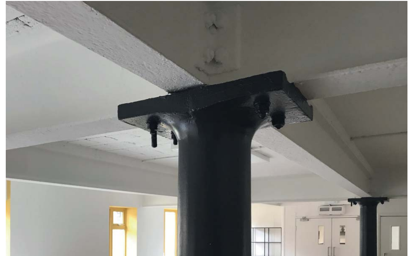
3.2.14 Existing exposed structure in office space on first floor
