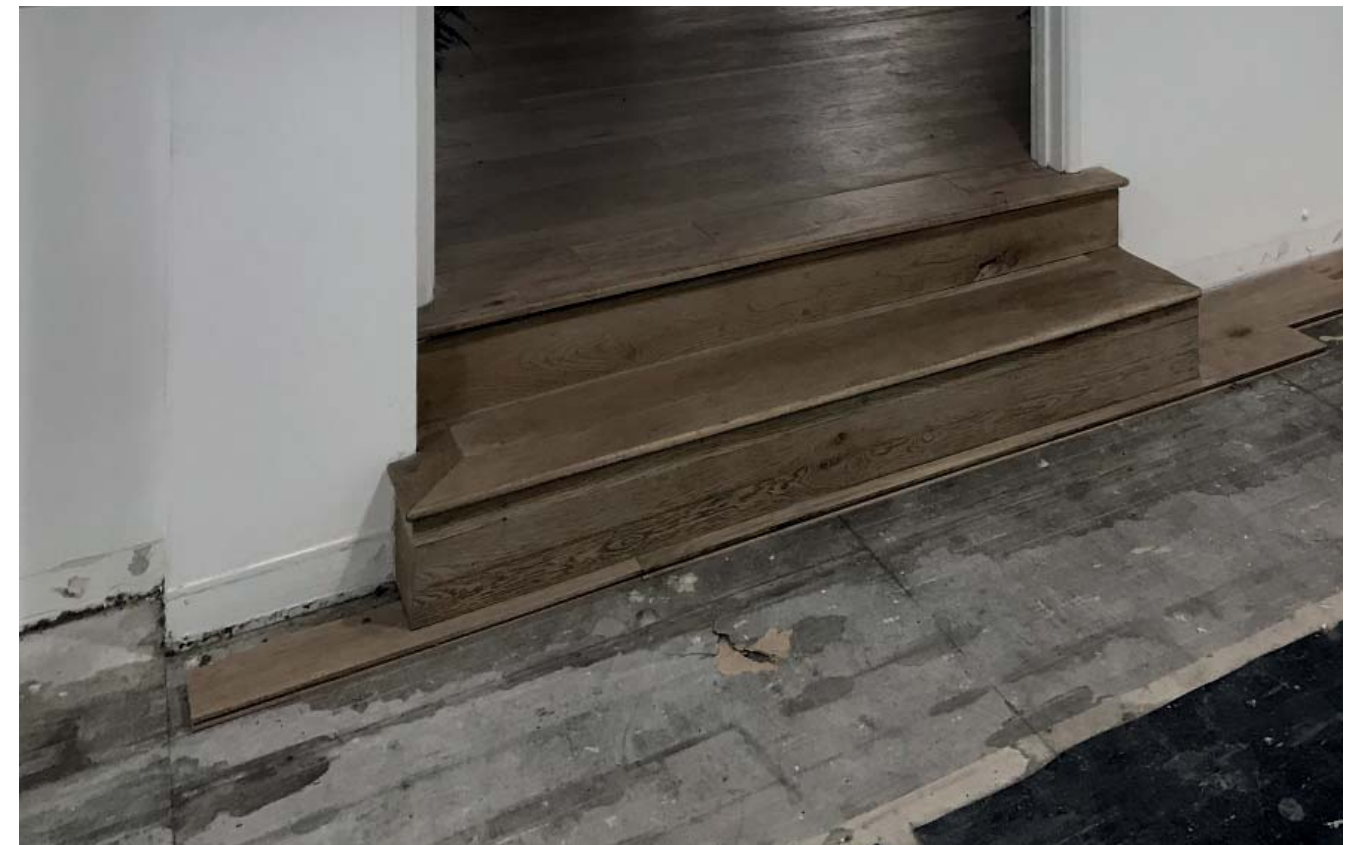
3.2.15 Existing raised floor in office space on first floor
