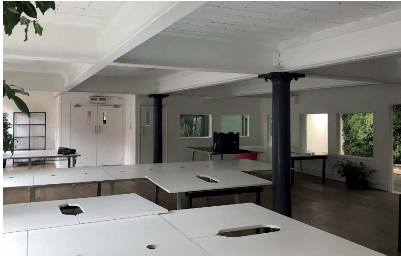
3.2.12 Existing office space on first floor
