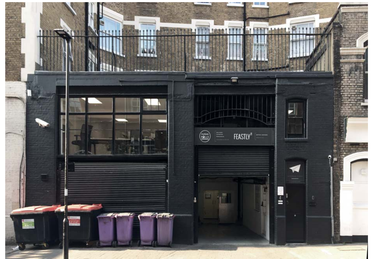
3.2.5 8-10 Warner Street - existing front elevation
