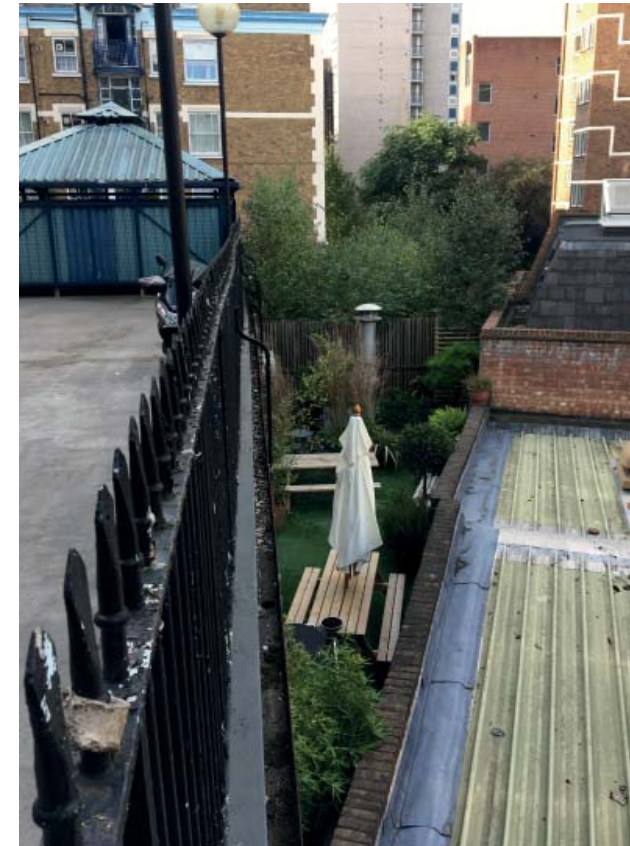
3.2.21 Existing terrace to rear
