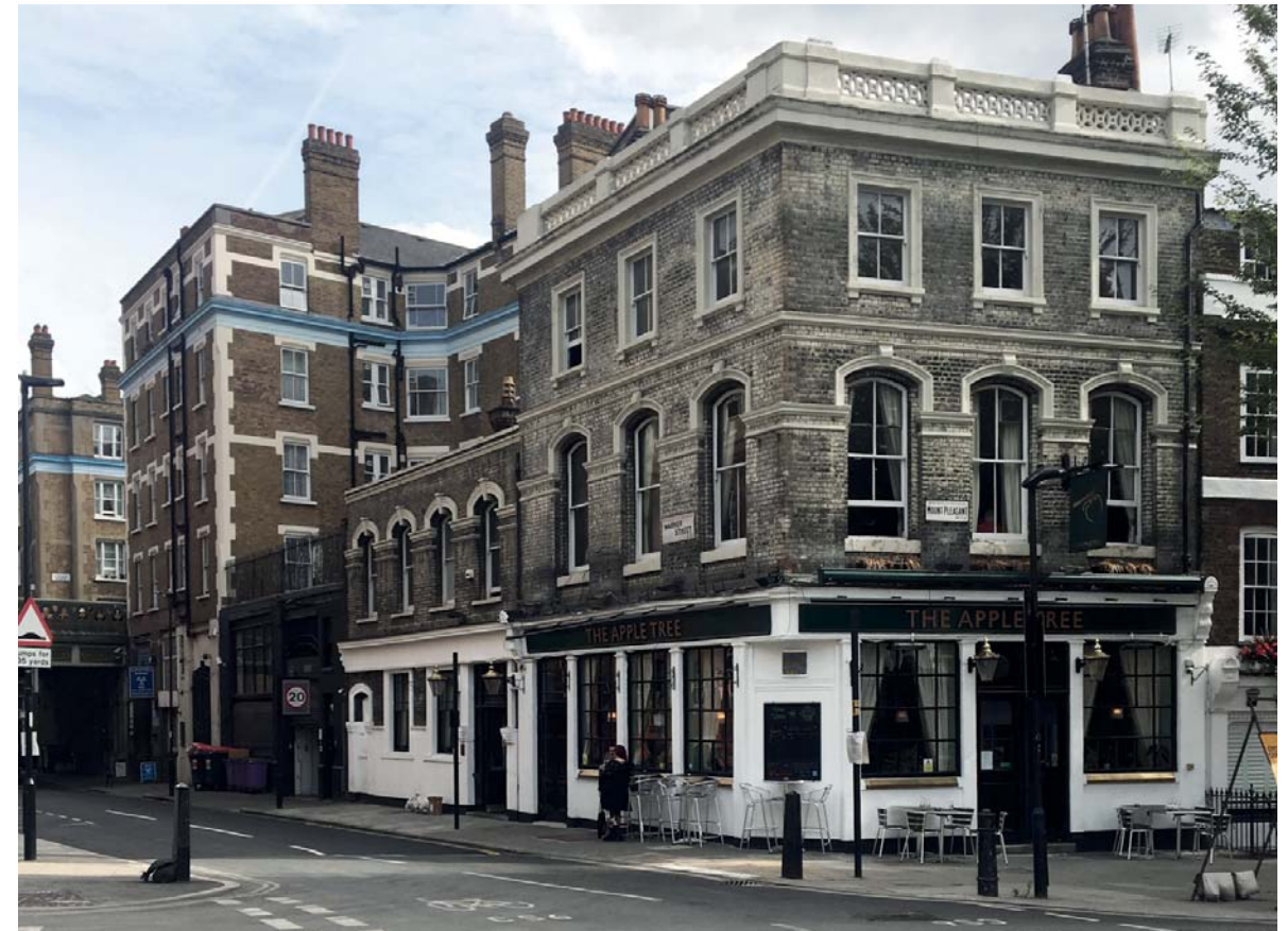
3.2.4 View looking east down Warner Street
