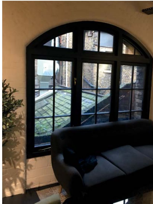
3.2.16 Existing window to courtyard to west
