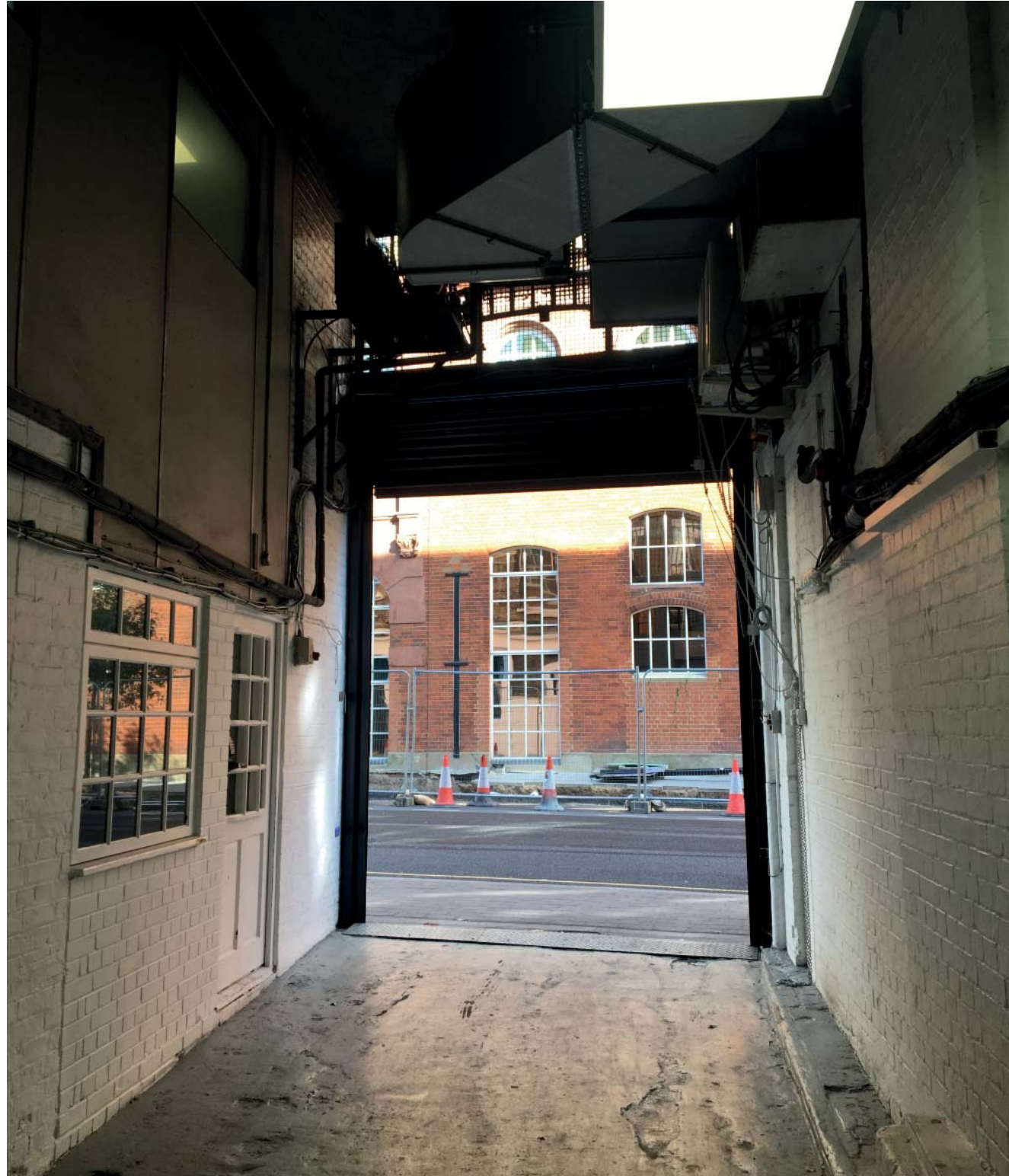
3.2.6 Main entrance from Warner Street
