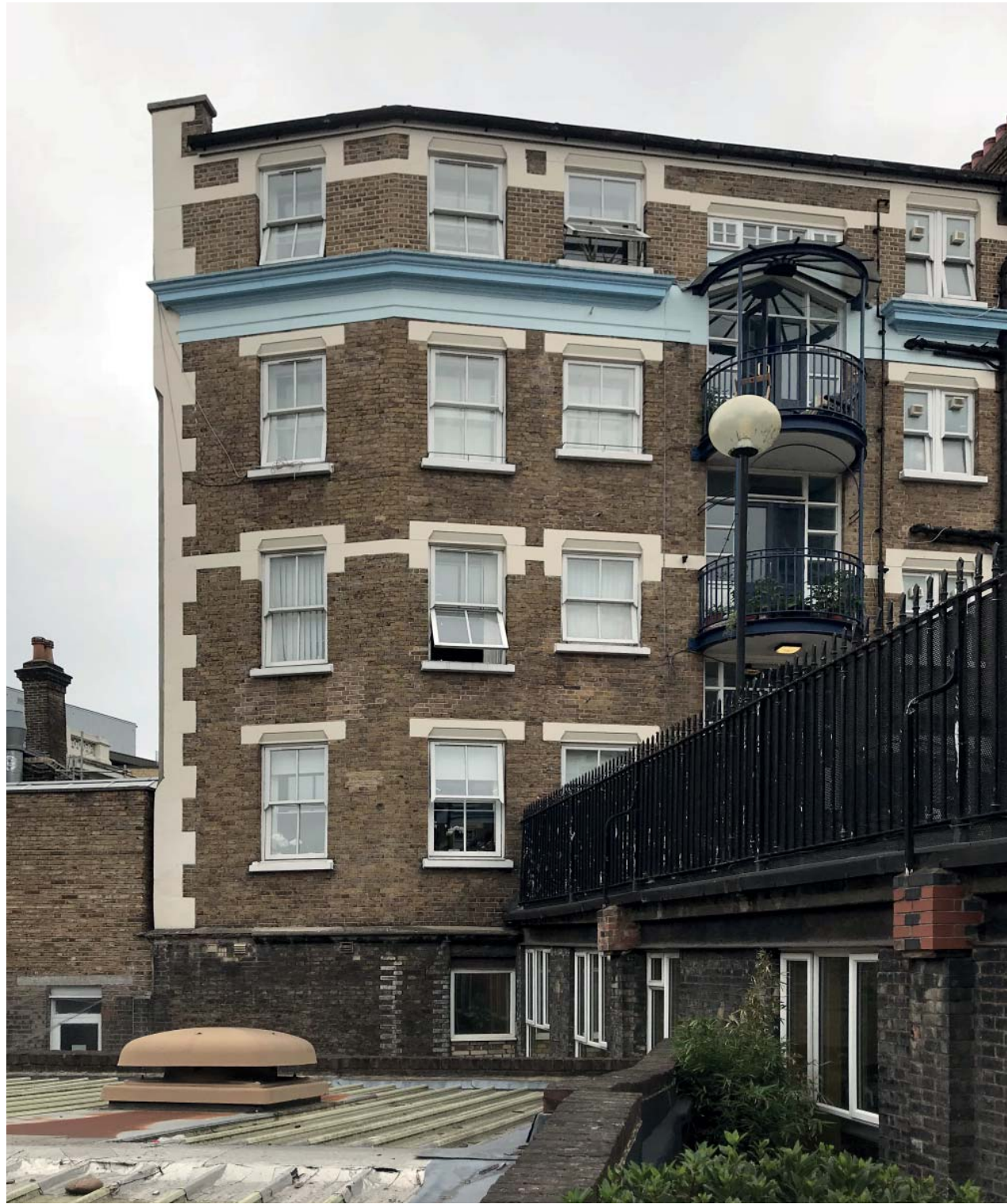
3.2.20 Existing building above site at rear
