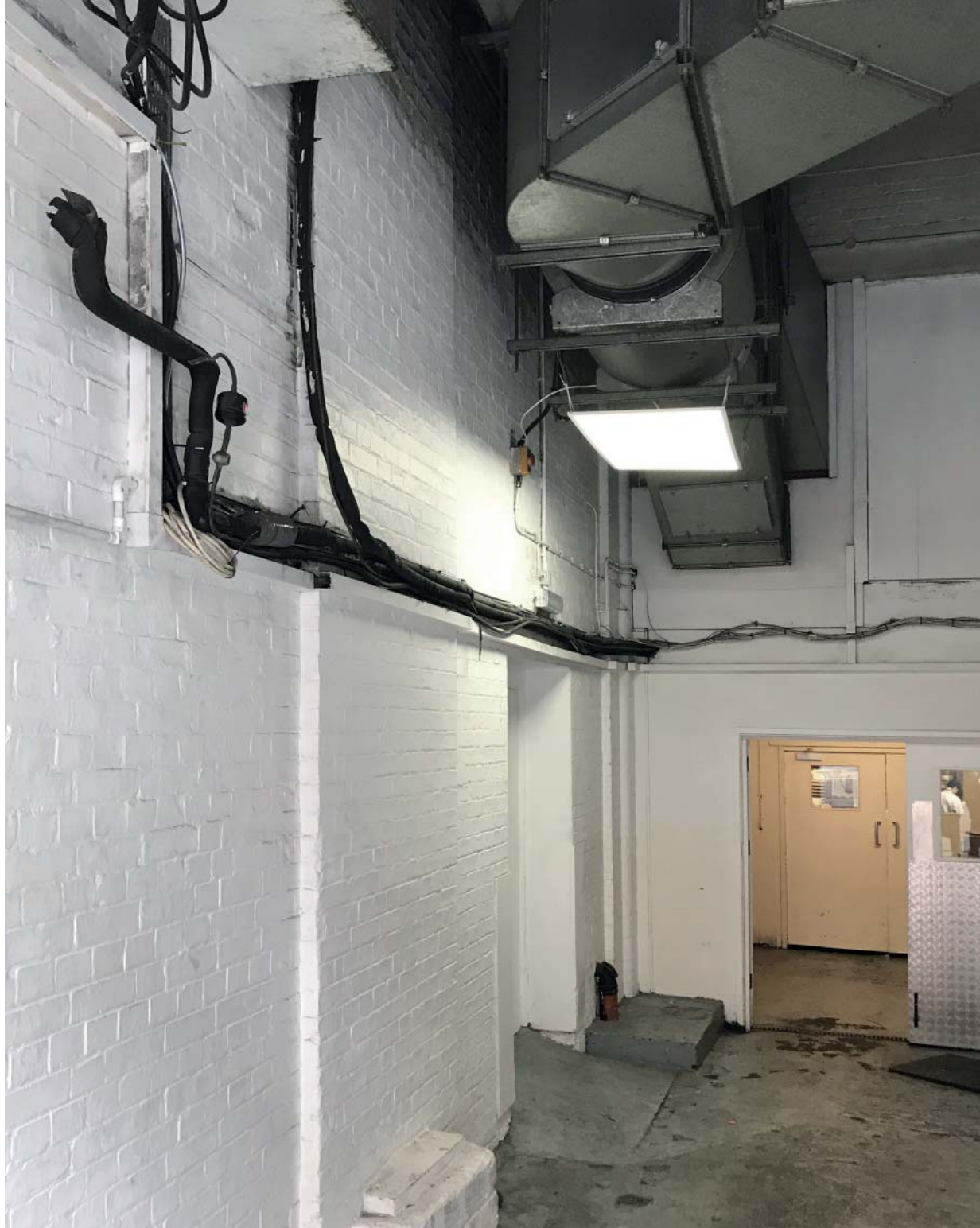
3.2.8 Main entrance from Warner Street
