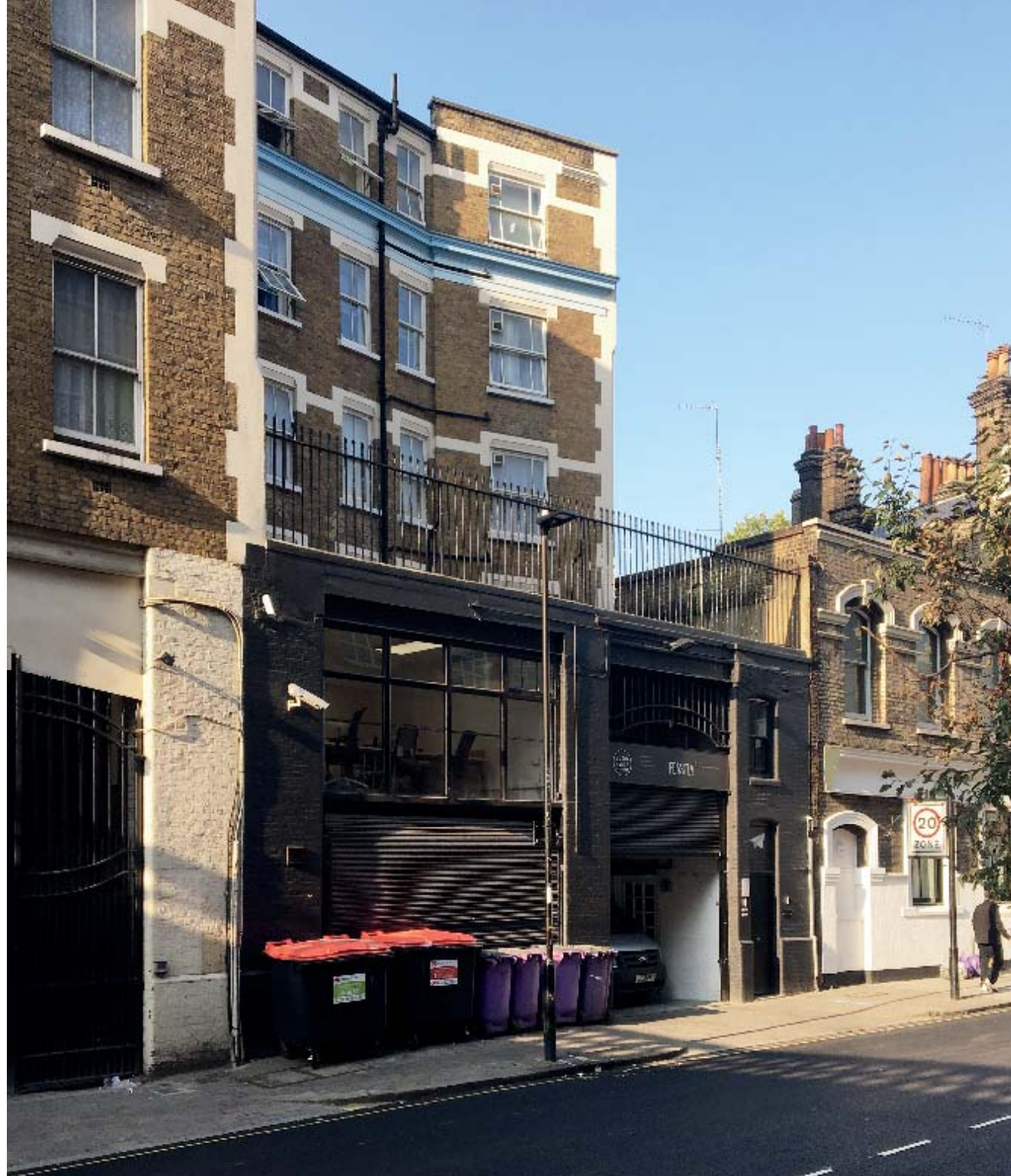
3.2.3 View looking west down Warner Street
