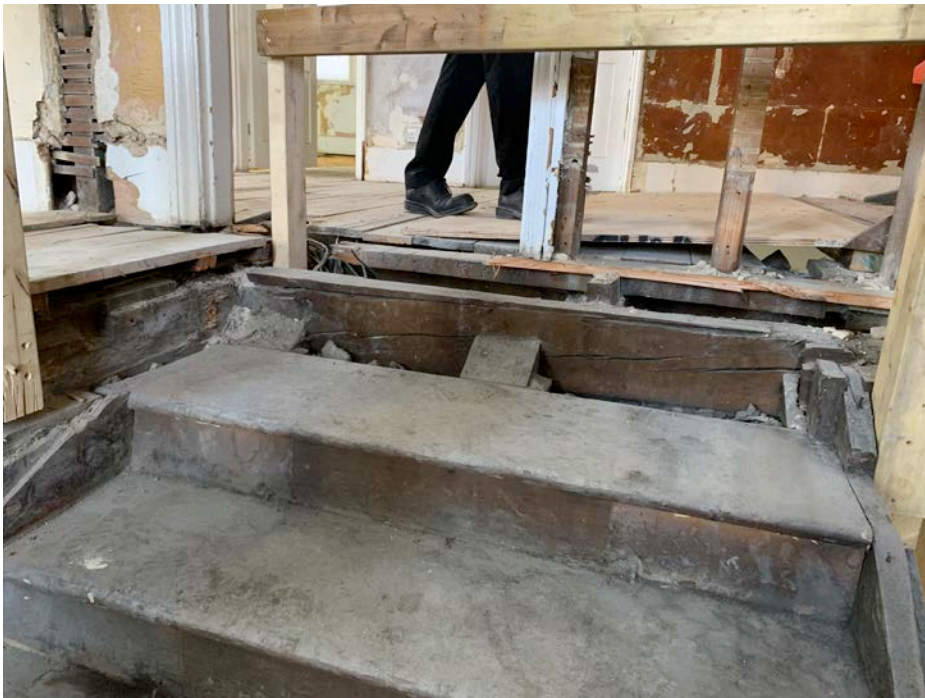
Detail showing raised landing floor is higher than arrival point of flight 2
