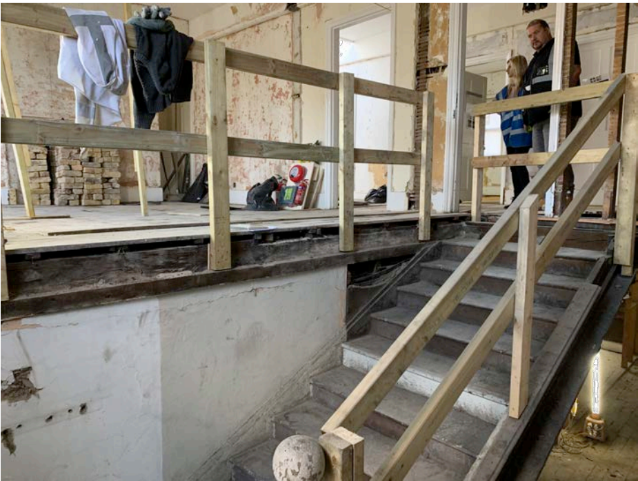
Original lateral floorplate trimmer to be retained. Wall to be repaired
