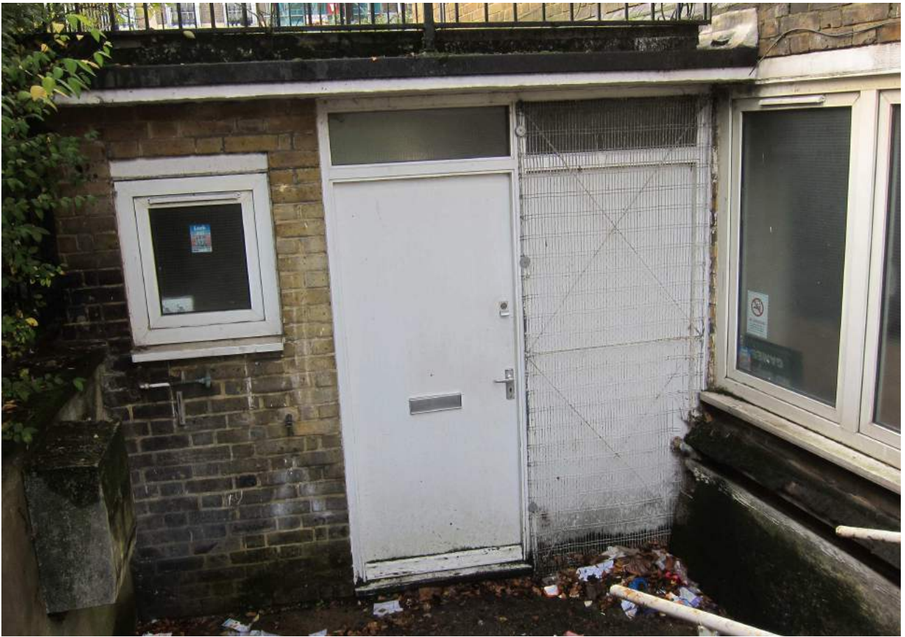
Existing entrance door and glazed screen (painted) from steps down
