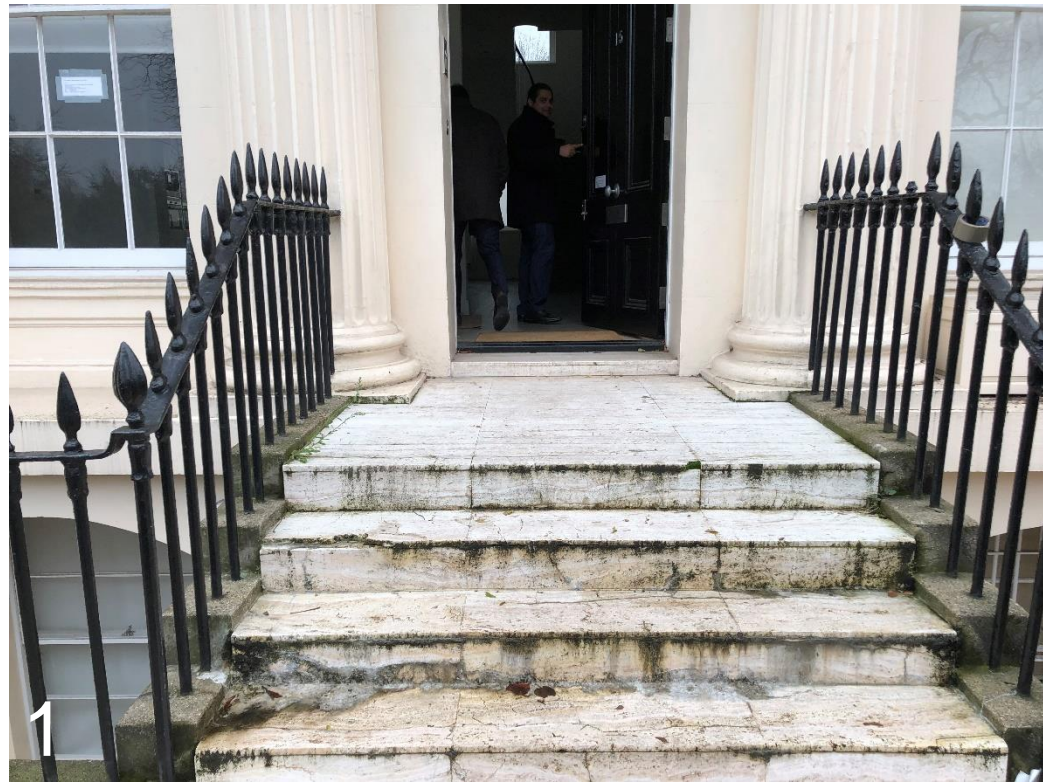
1 Existing steps from street level to ground floor level
