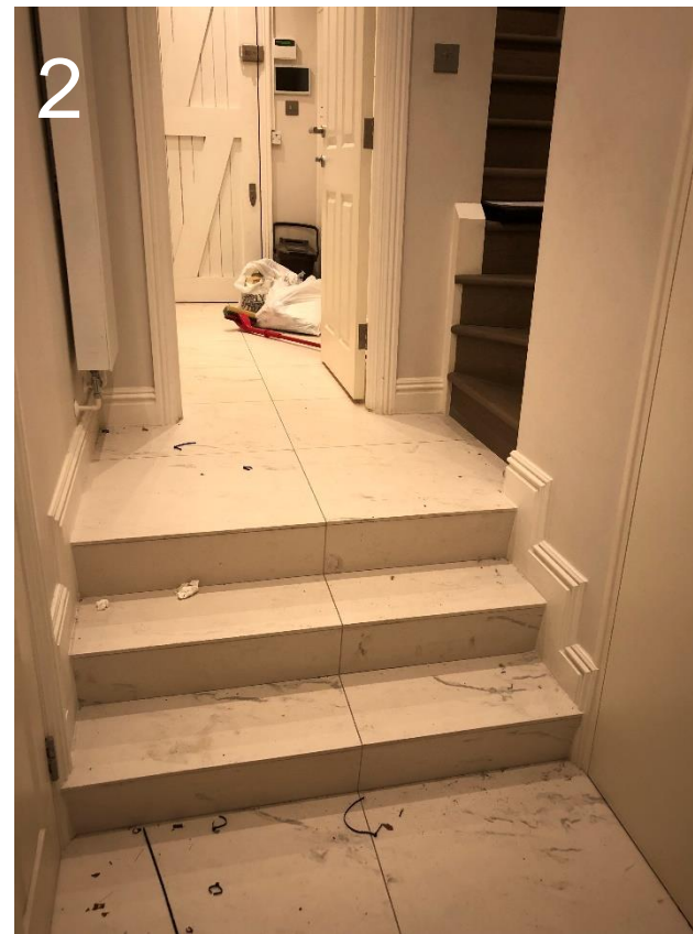
2 Existing Steps leading up to Utility room and garage level
