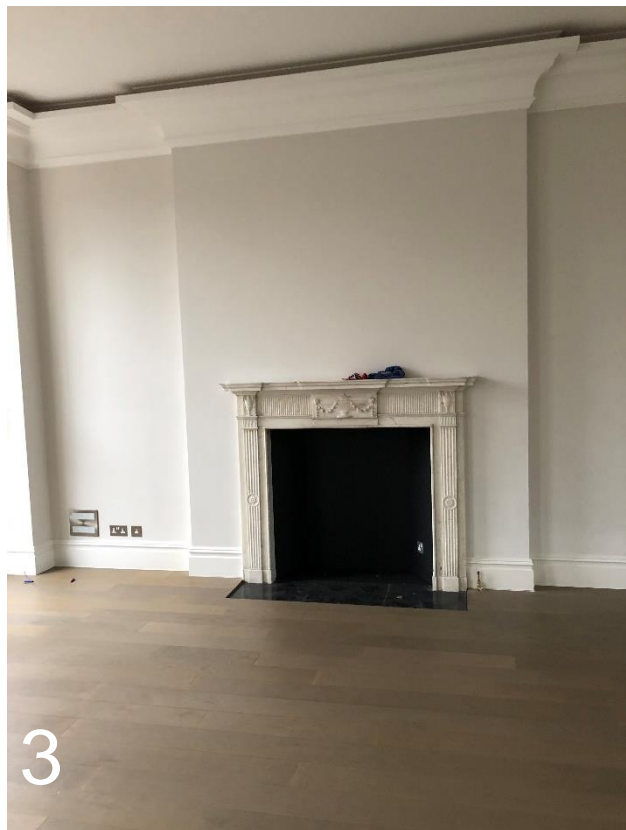
3 Existing fire place in Living room
