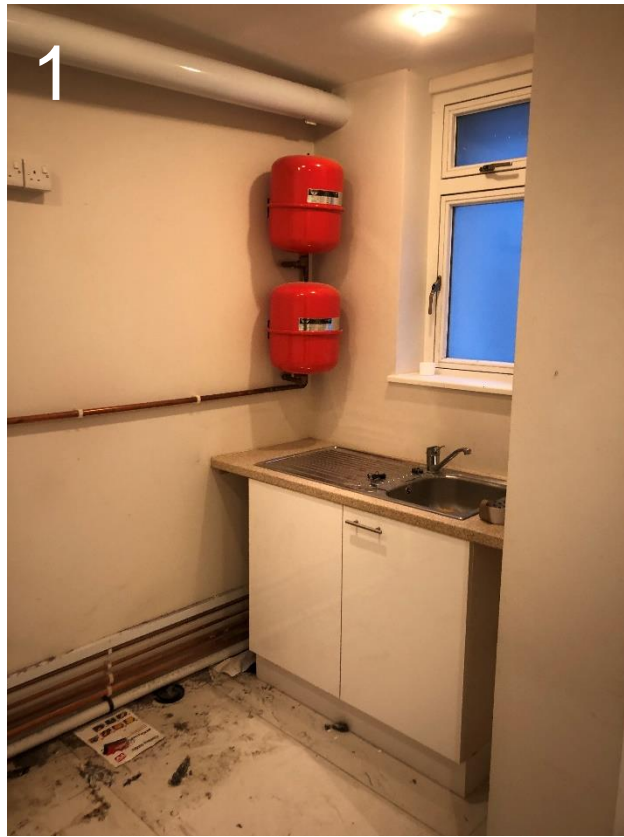
1 Utility room, View of existing sink and rear window.
