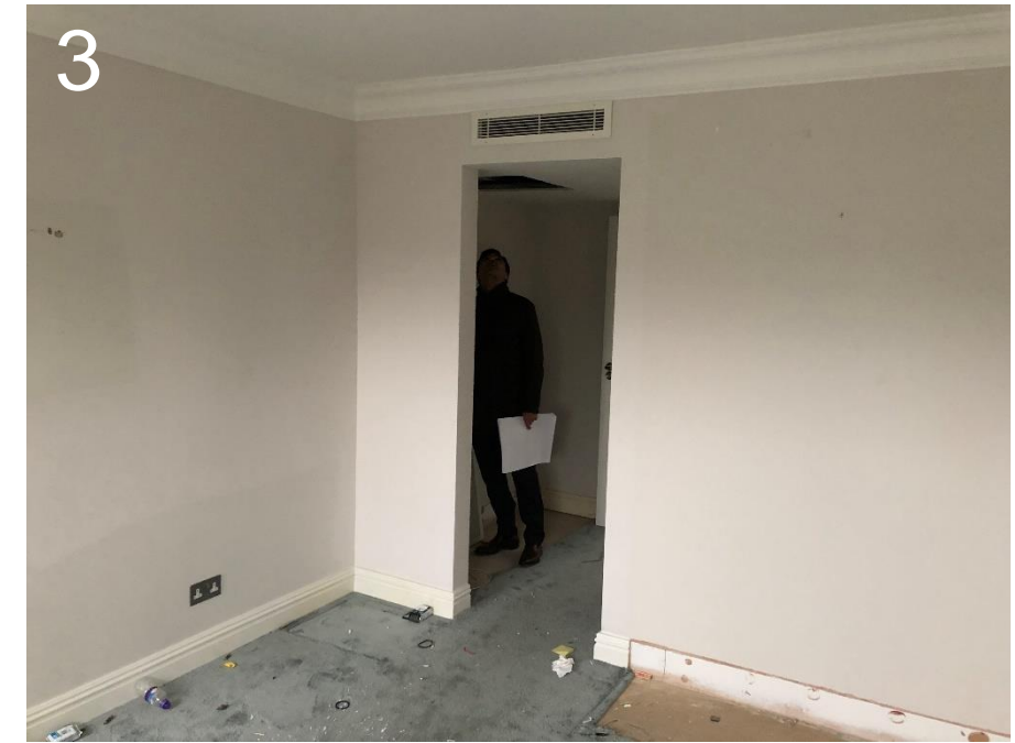
3 Existing opening into bedroom 4
