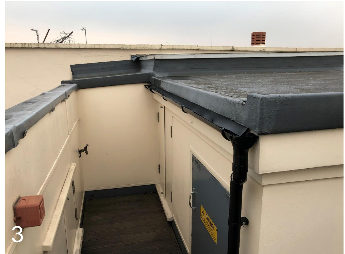
3 Existing lower level of Roof Terrace with access to storage cupboards
