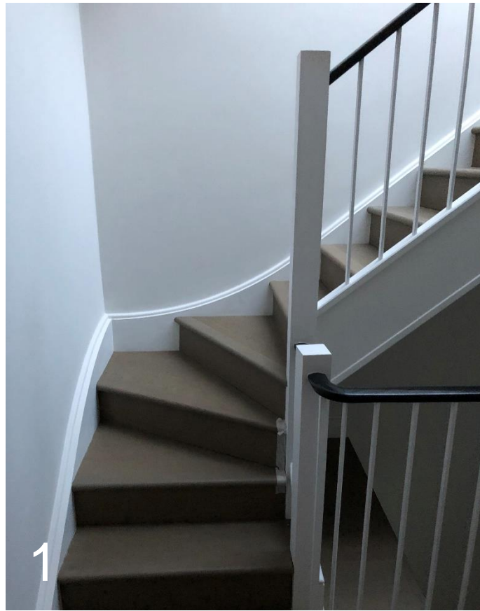
1 Existing winding staircase to Roof Terrace
