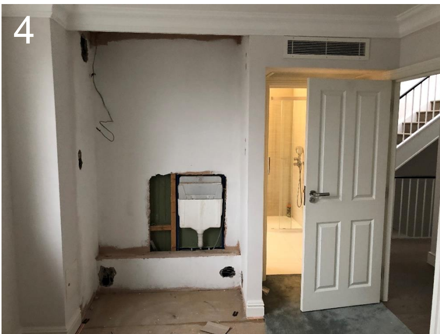
4 Existing En-suite for Bedroom 2
