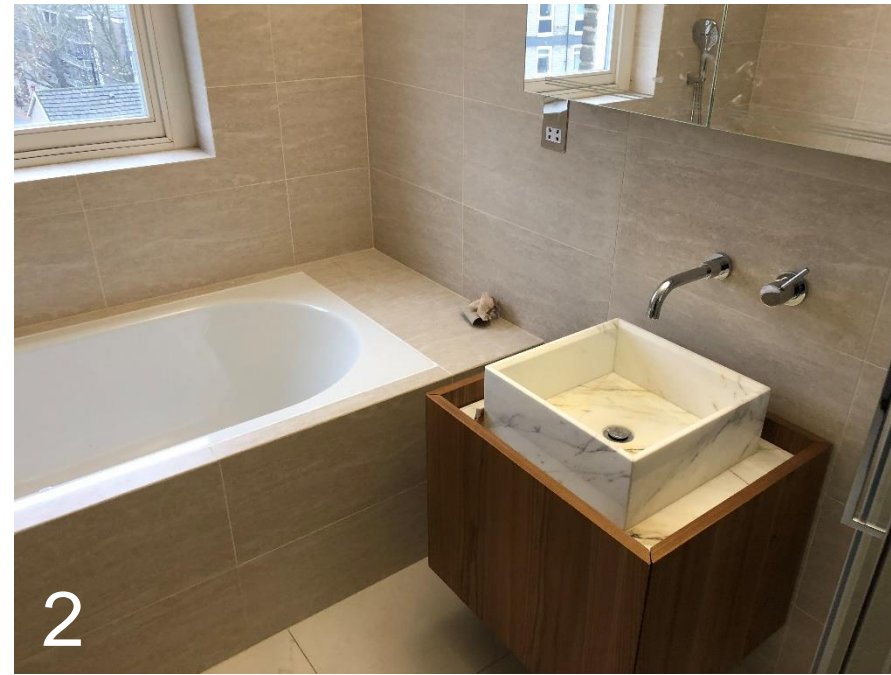
2 Existing En-suite for Bedroom 2
