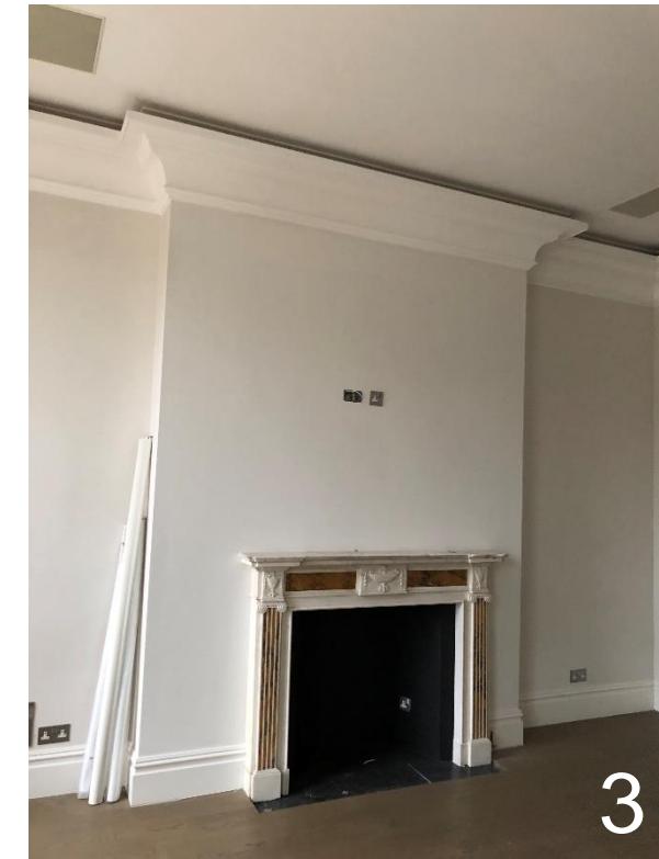
3 Existing fire place in dining room
