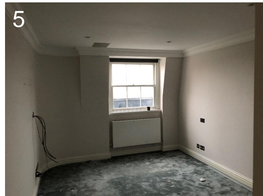
5 Existing Bedroom 3 with curved wall and dormer
