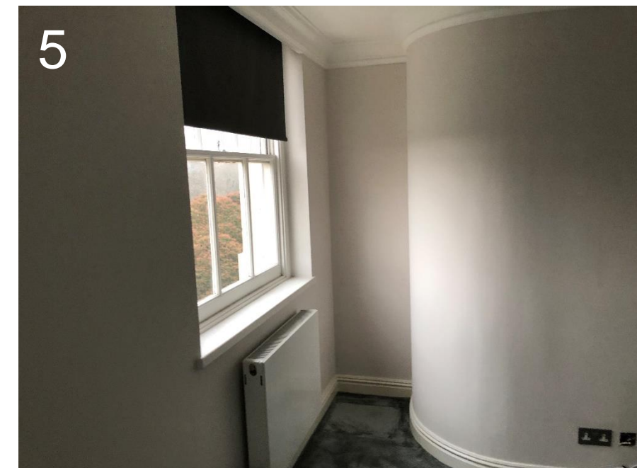
6 Existing curved wall with dead space in Bedroom 4
