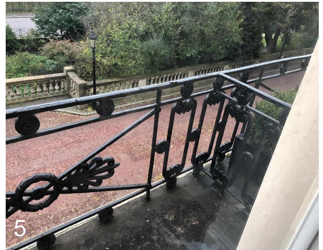
5 Existing balcony (no access)
