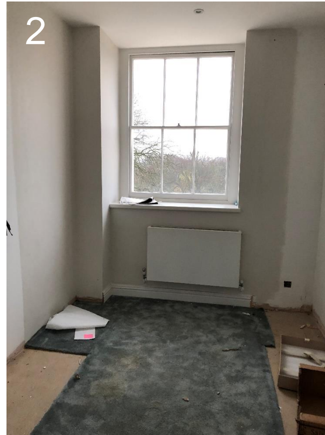
2 Existing Dressing Room for Master Bedroom
