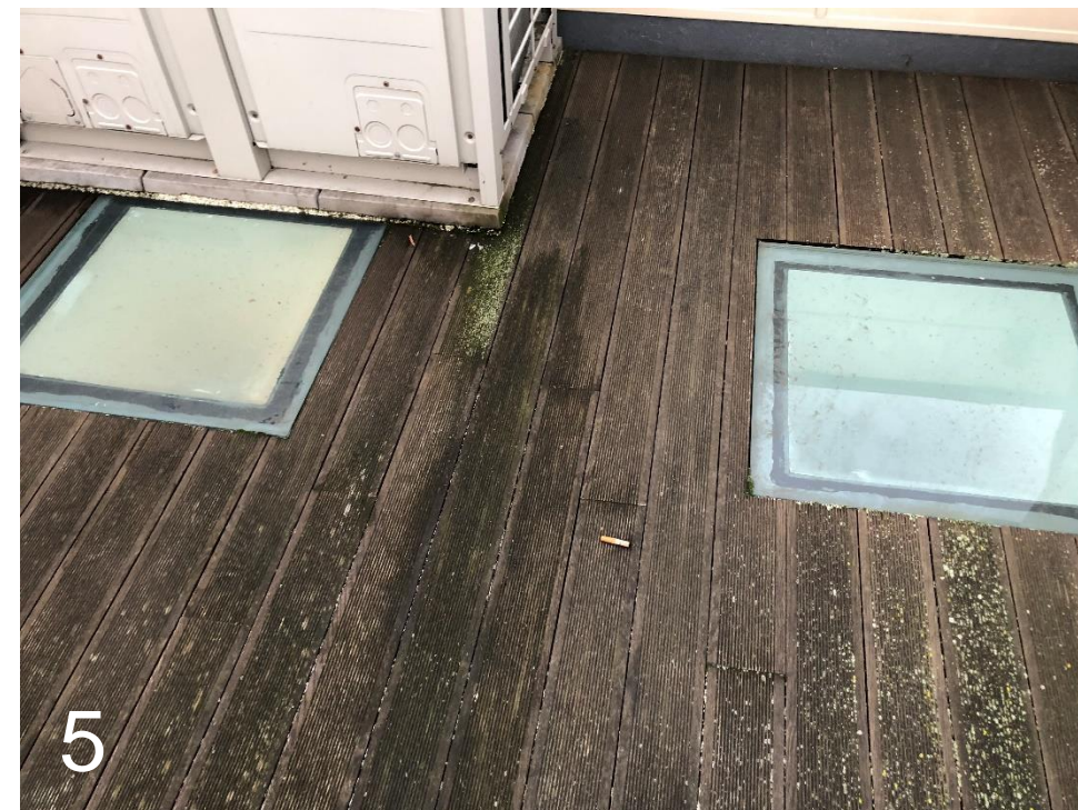
5 Existing rooflights on timber deck
