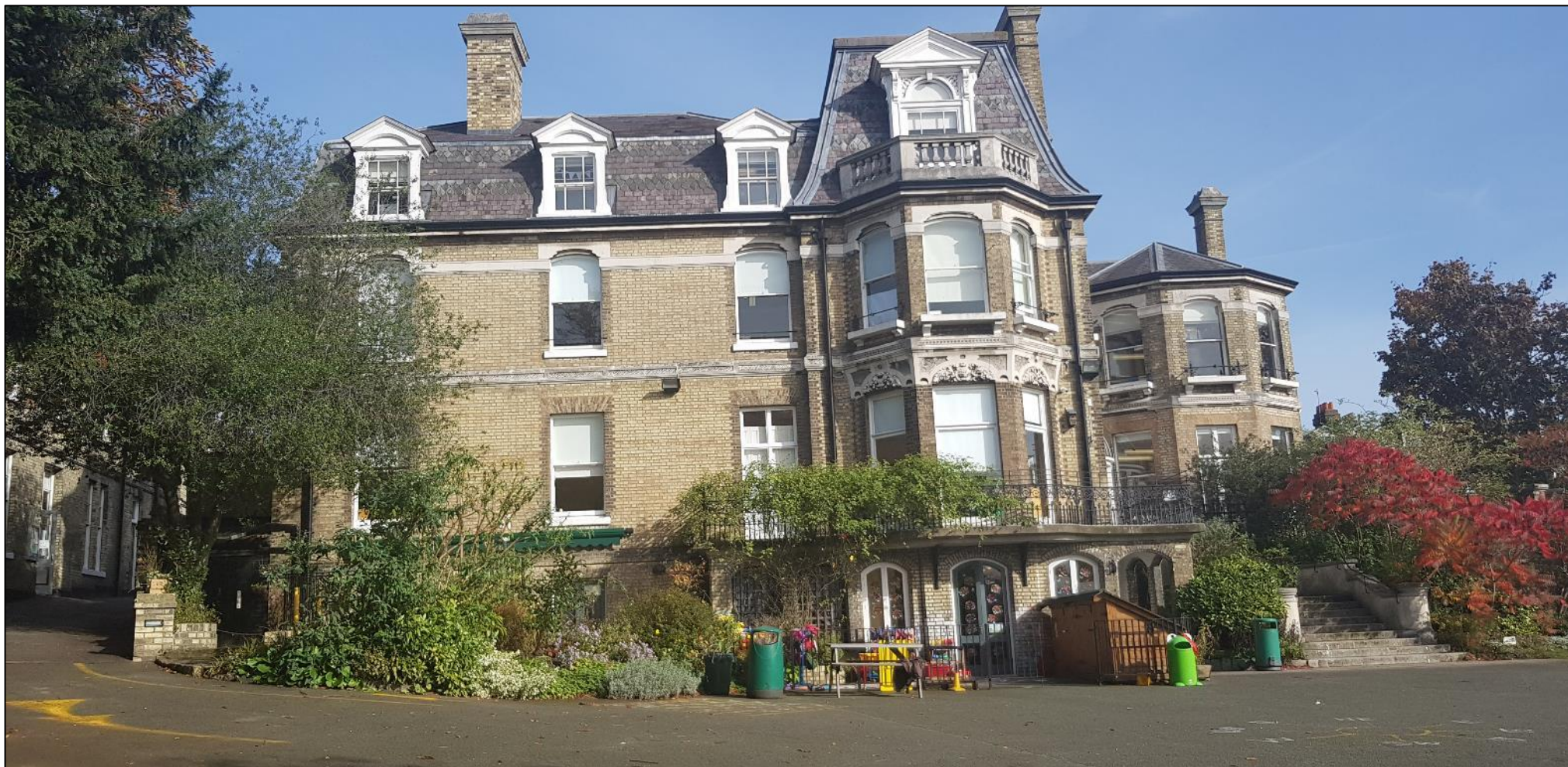
Photo 2: Looking north at the rear B1.
