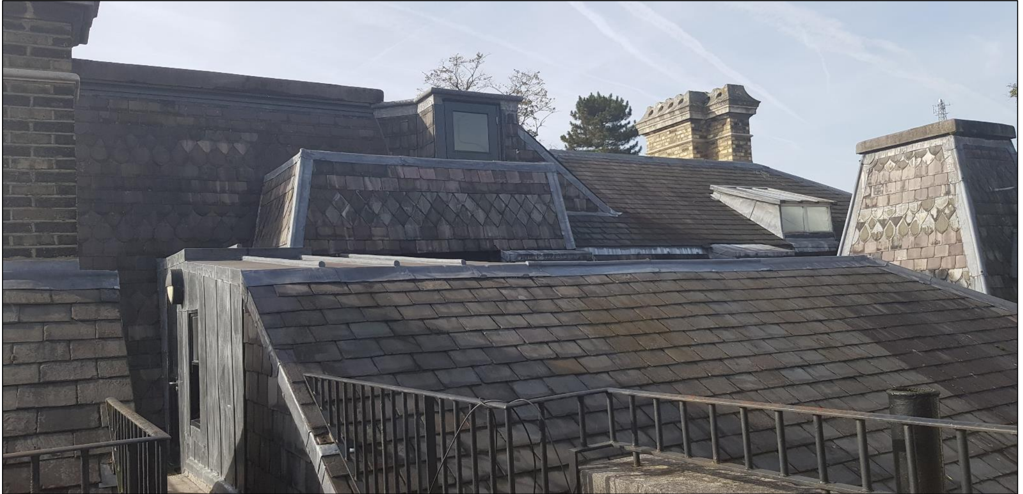
Photo 4: The roof of B1.
