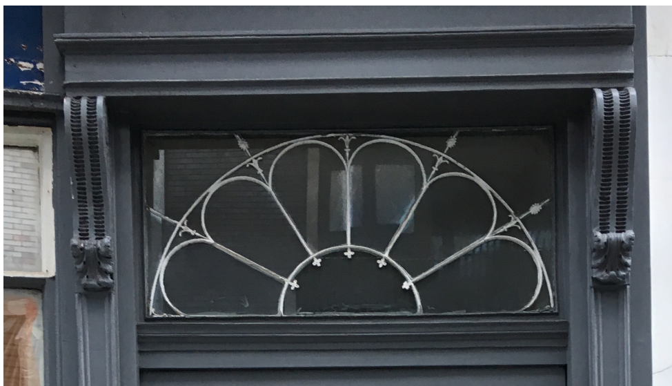
Original fanlight at No 20 Cleveland Street, with original timber consoles
