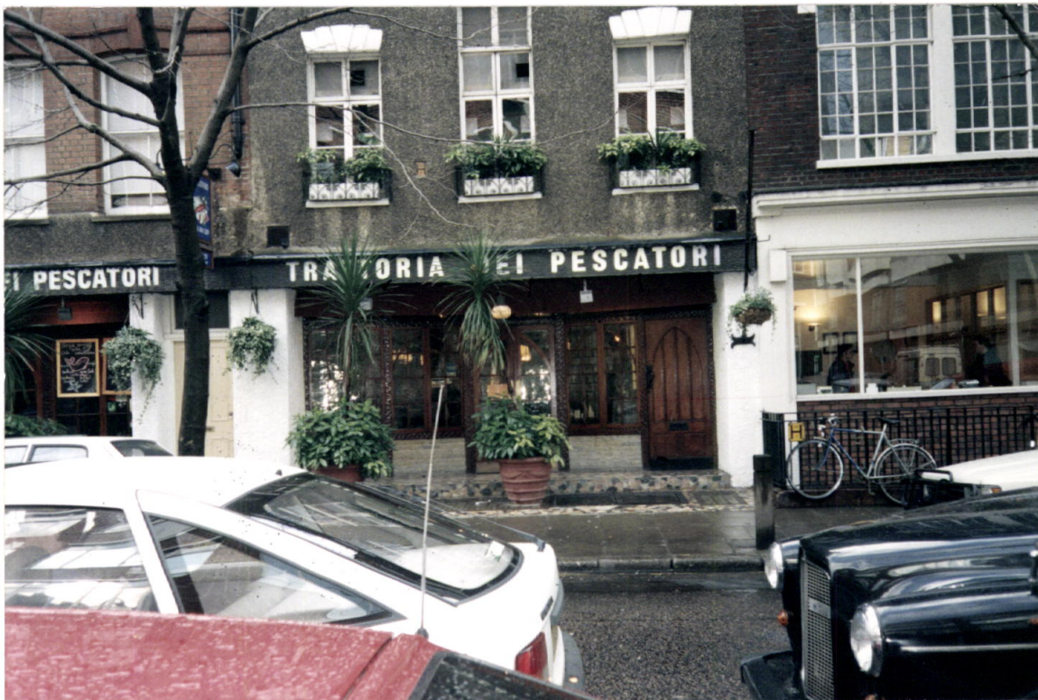
EXISTING SHOP FRONT—No. 57 CHARLOTTE ST. W1
