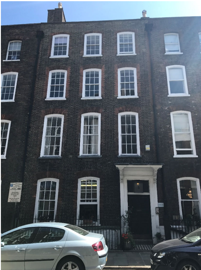
Fig 1 Street View: 5 Great James Street
