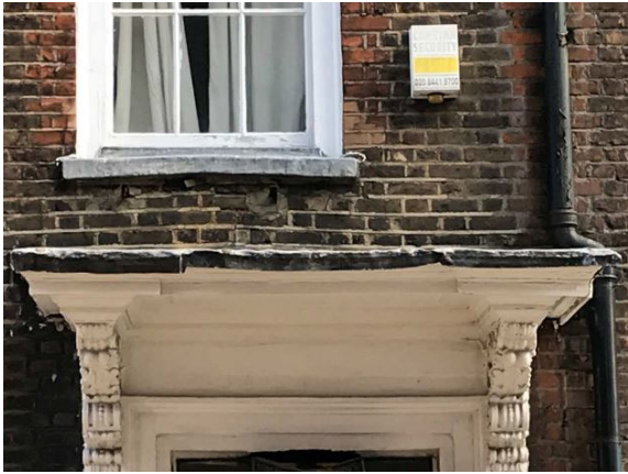
Fig 10 Front door canopy lead repairs.
