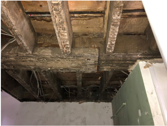
Fig 3 Existing failing timber floor beam that requires strengthening.
