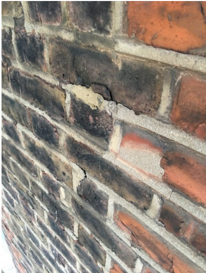
Fig 6 Close up of failing historic repointing.
