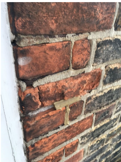
Fig 5 Close up view of poor historic repointing around window reveals
