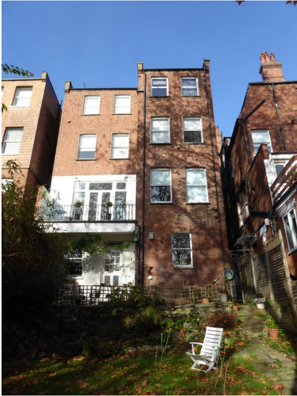
Photo E: View of the rear elevation of the application site
