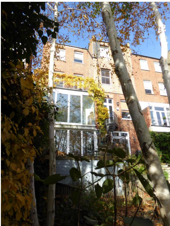
Photo G: View of the rear elevation to the neighbouring property at no. 6 Froggnal Lane
