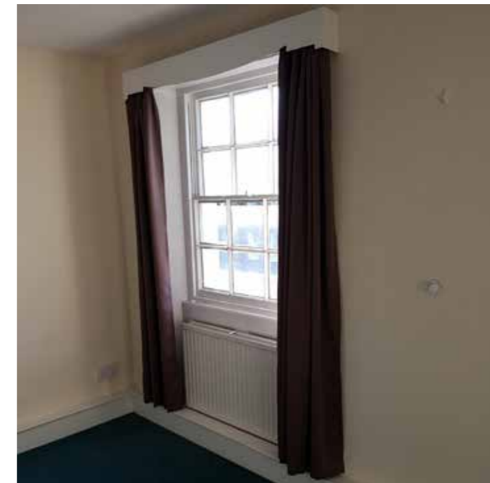
15 - Services in boxed skirting. Late addition window pelmet to omit
