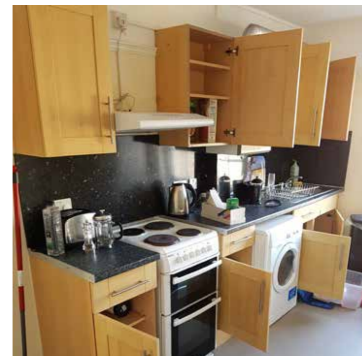
16 - Existing low quality kitchen units
