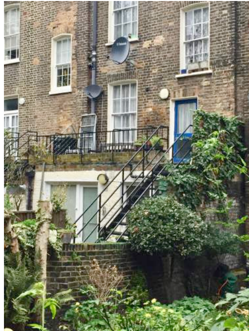
No. 15: Black metal access stair from rear terrace to garden (view from garden of No. 11)
