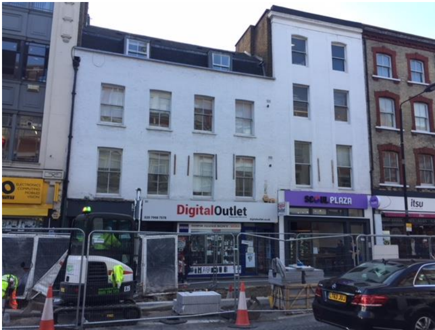
Photo 1 (above): Front elevations of Nos. 51 and 52 Tottenham Court Road
