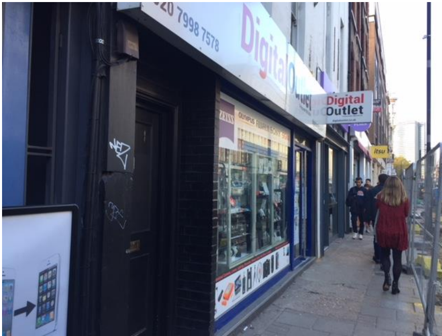
Photo 3 (above): Close up view of shopfront at No. 51 Tottenham Court Road looking north
