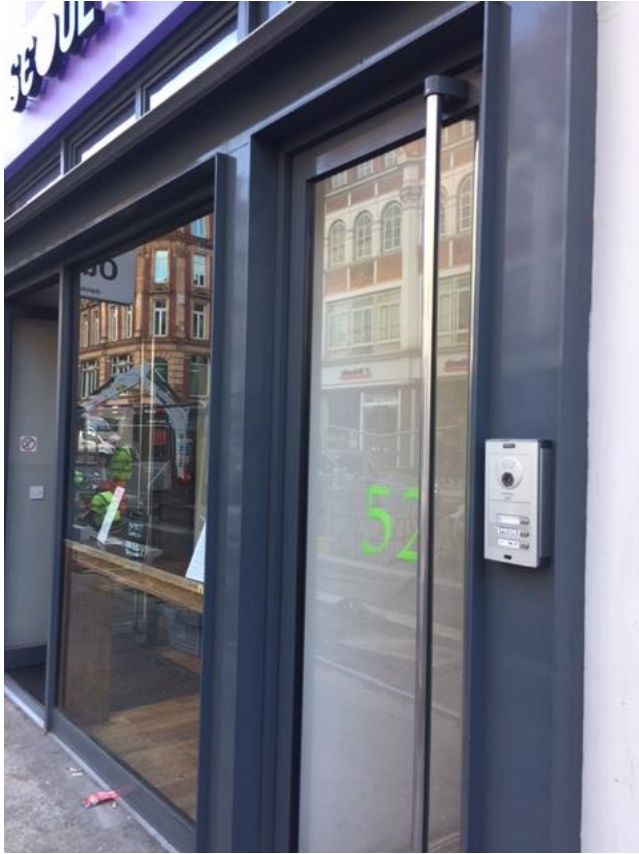
Photo 7 (above): Close up view of shopfront at No. 52 Tottenham Court Road including door to offices above
