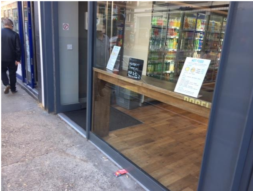
Photo 6 (above): Close up view of shopfront at No. 52 Tottenham Court Road
