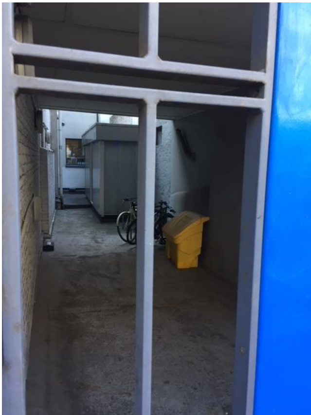
Photo 8 (above): View of access road adjacent to ground floor of No. 51 Tottenham Court Road with first floor of building above
