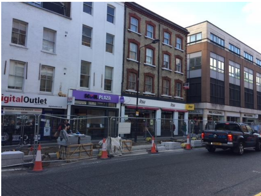
Photo 2 (above): Front elevations of Nos. 51, 52, 53 and 54 Tottenham Court Road
