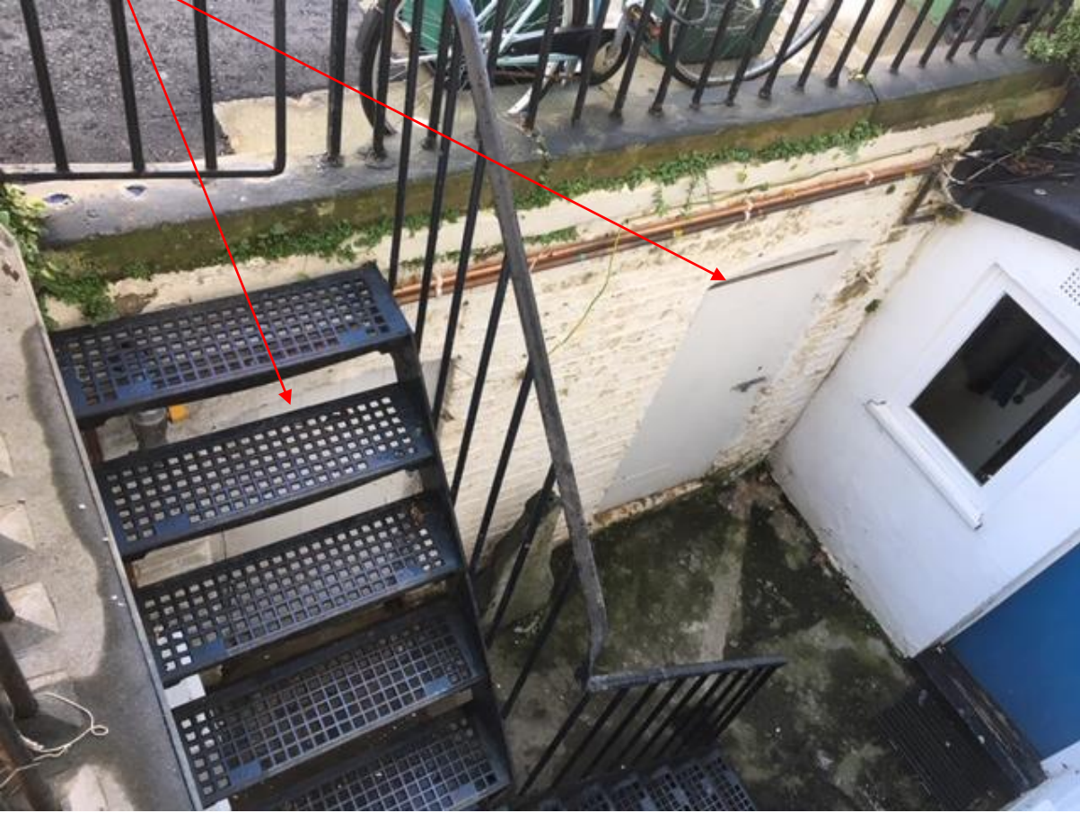
Photo 3 (below): Existing vault doors
