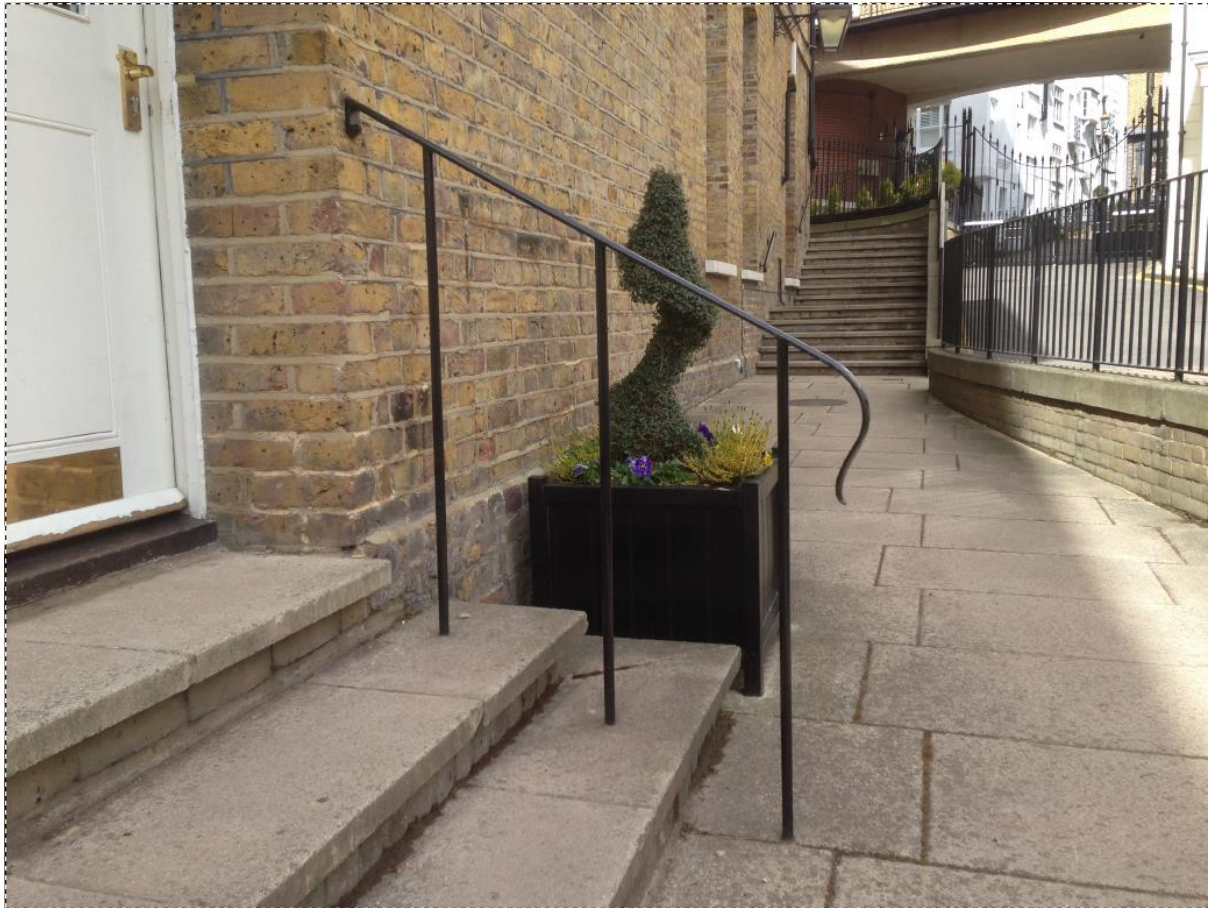
Photo 2 (above): Design of the handrail at Old Upper Hampstead walk.
