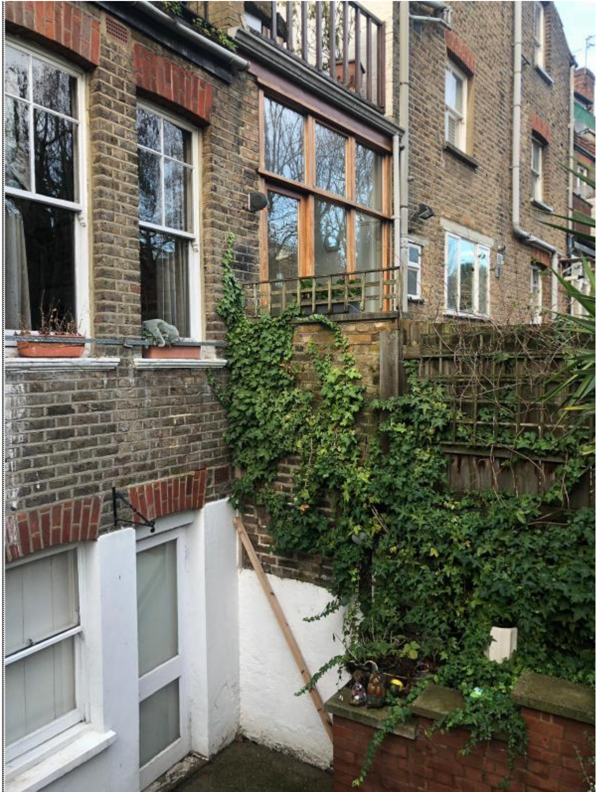
Photo 4 (above): View of side boundary shared with no. 33 Dennington Park Road
