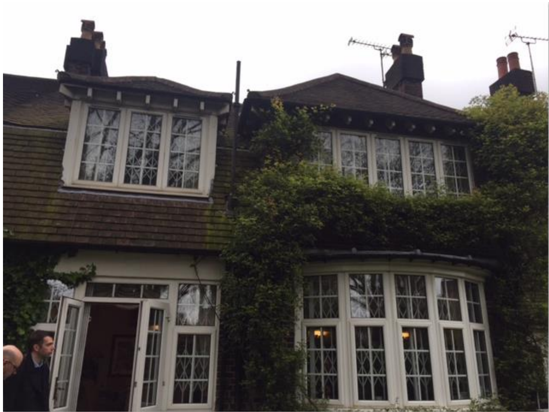
Photo 5 (above): Front elevation
