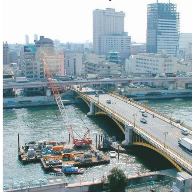
Seismic Reinforcement Work on Bridge Foundation
