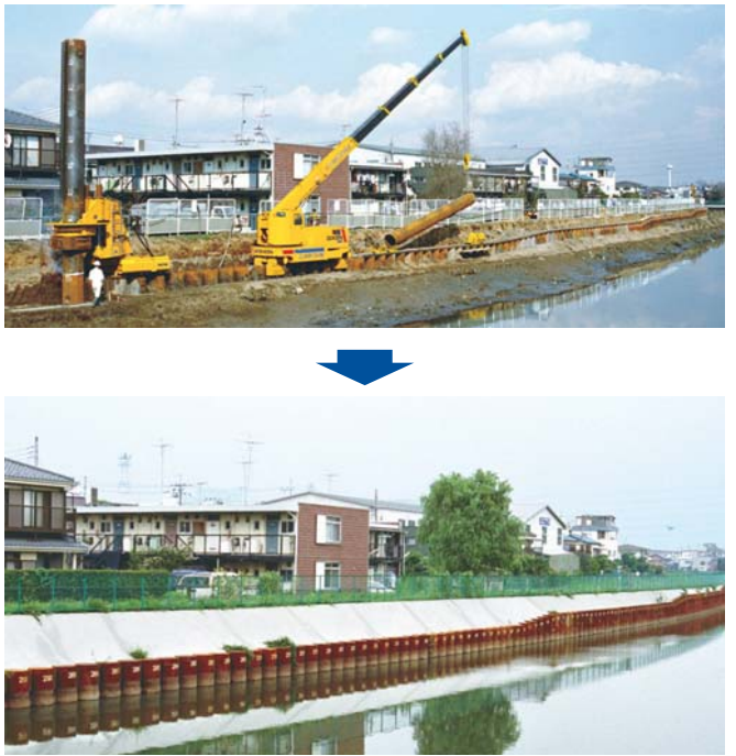
Build up Implant Structure Bank Protection with Kasetsu-less Construction
