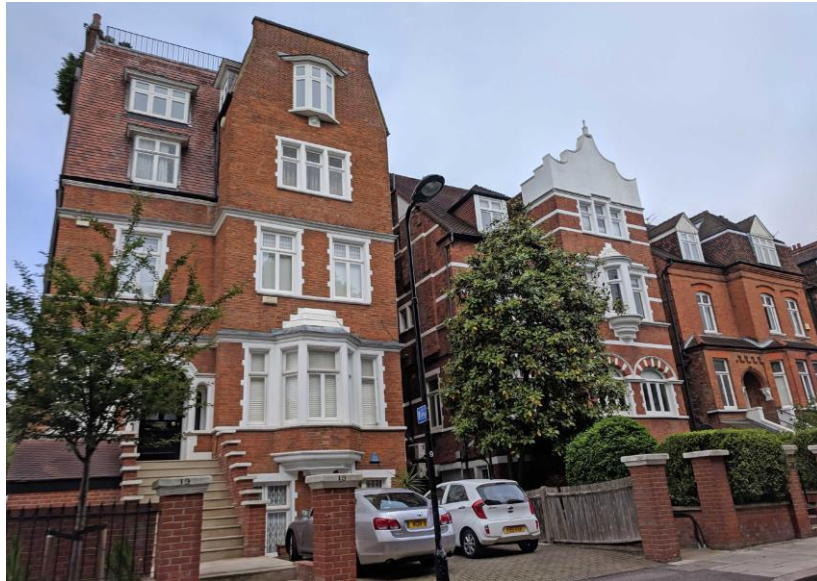
21 Maresfield Gardens as Existing (view from the southeast)
