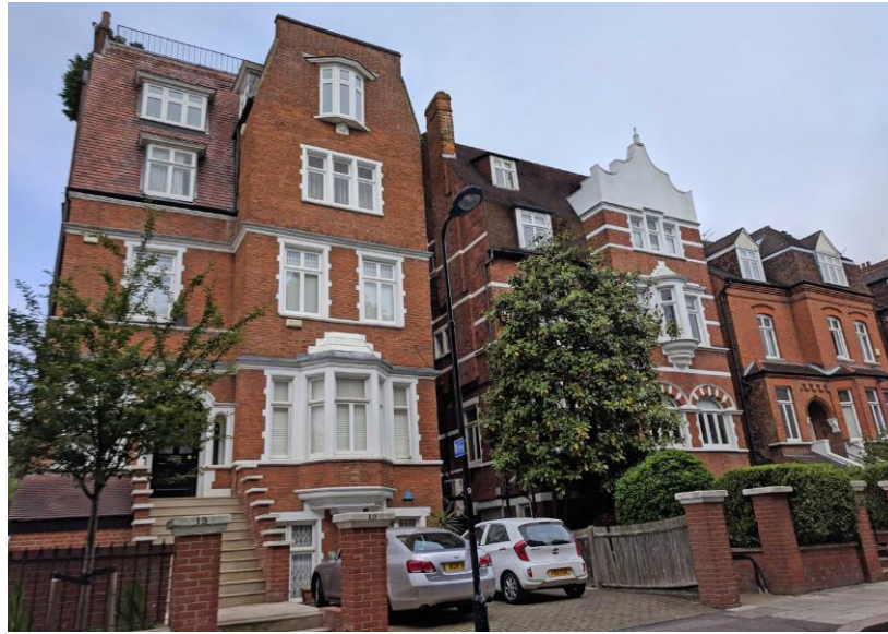
21 Maresfield Gardens as Proposed (view from the southeast). NB proposed dormer at third floor level has been omitted and replaced with a conservation type roof light
