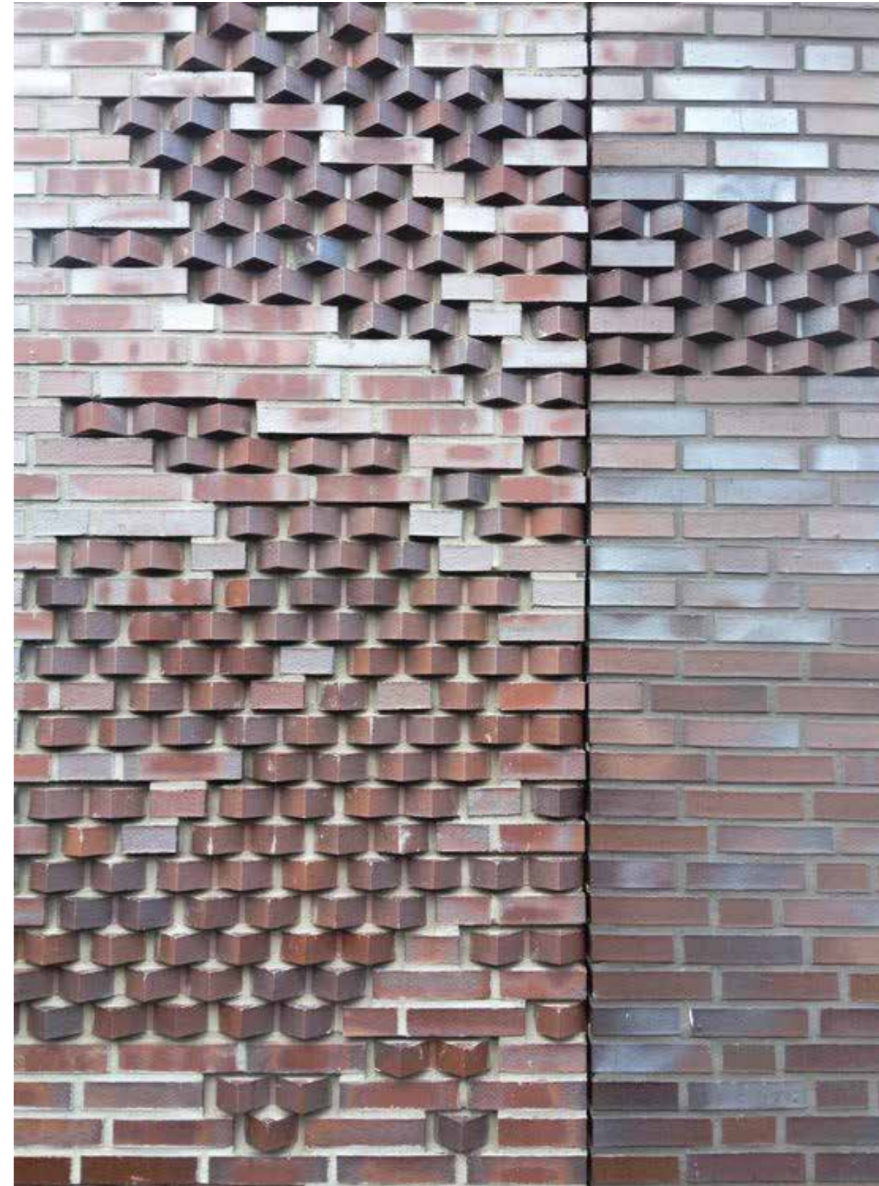
REAR OF 17 STRATFORD VILLAS PROJECT REFERENCES IMAGES NOT TO SCALE NW1 9SJ LONDON
