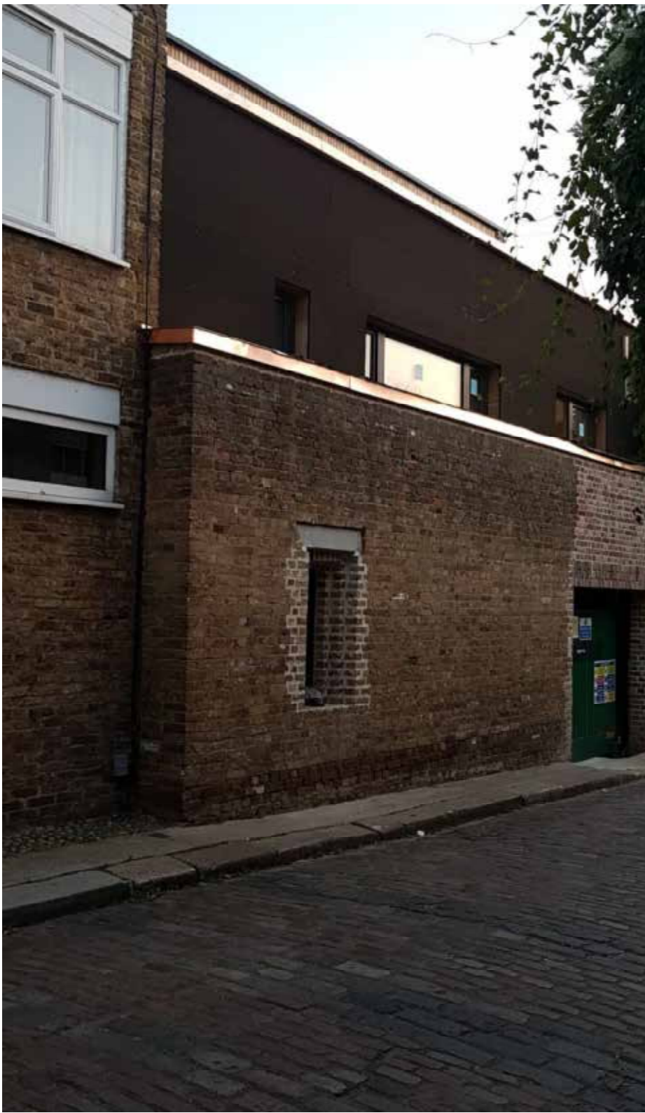
5 REAR OF 3 CAMDEN SQUARE
