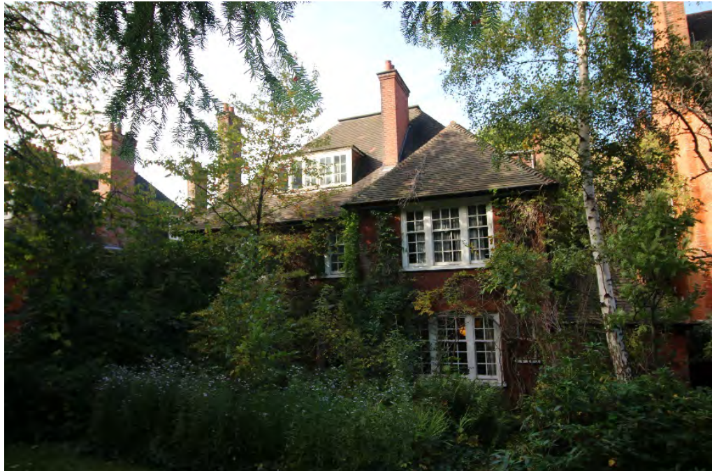
Figure 4: No. 24 Heath Drive, Rear (South East) Elevation, 2016
