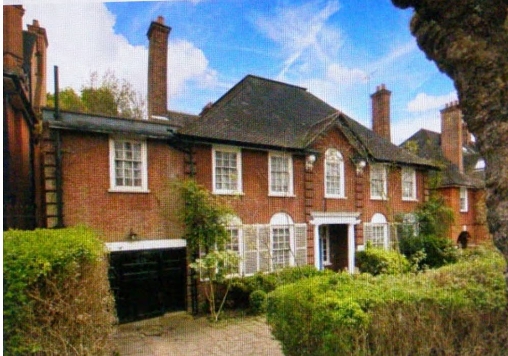
Figure 3: No. 24 Heath Drive, Front (North West) Elevation (2016)
