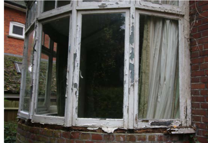
Current condition of the bay window
