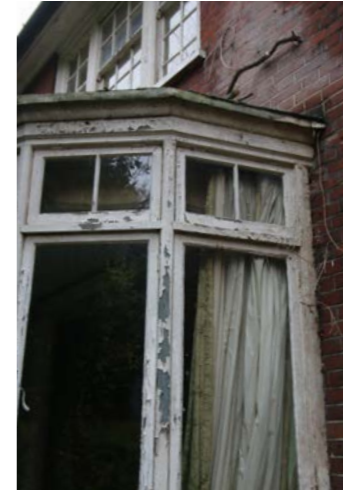
Current condition of the bay window
