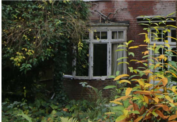
Rear View to the non-original bay window
