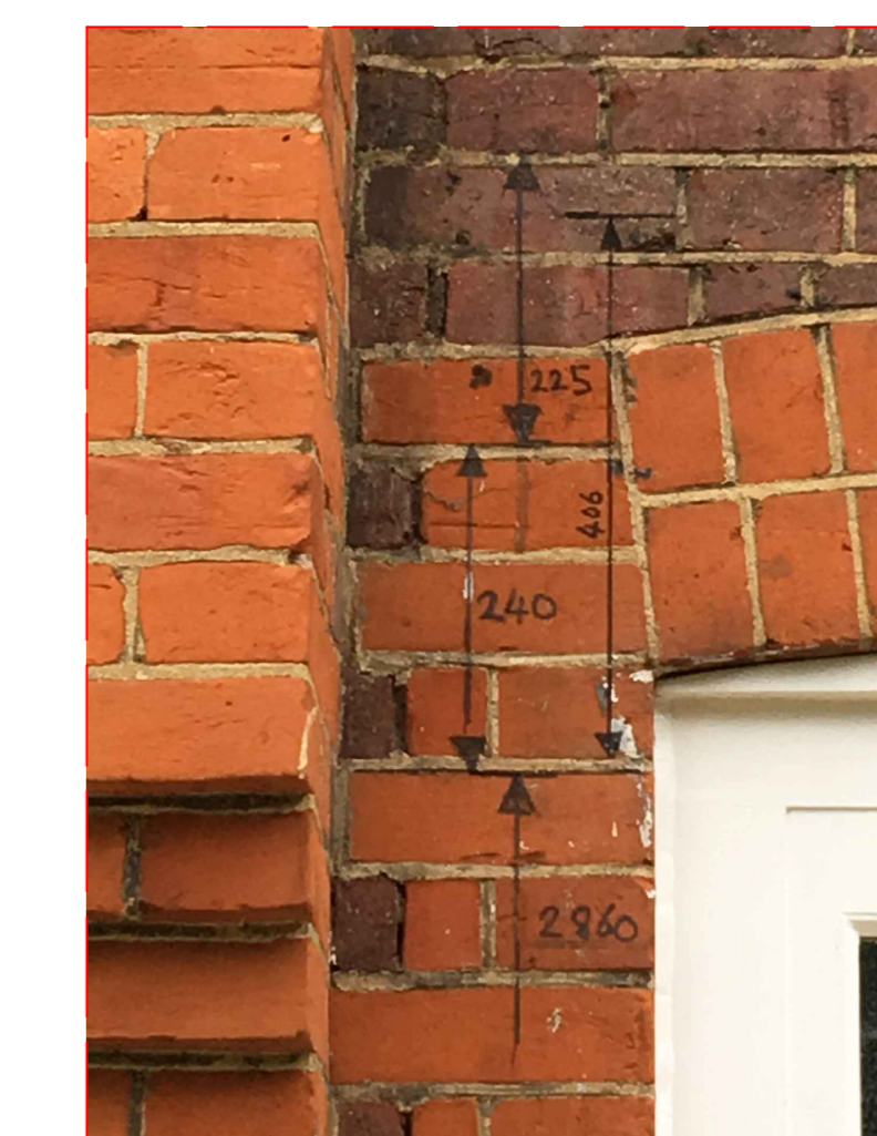
CONTRAST BRICKWORK DETAIL New brickwork to match
