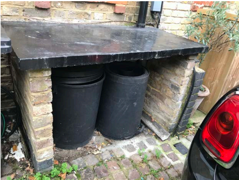
Photo 5 - Existing bin enclosure to be demolished.
