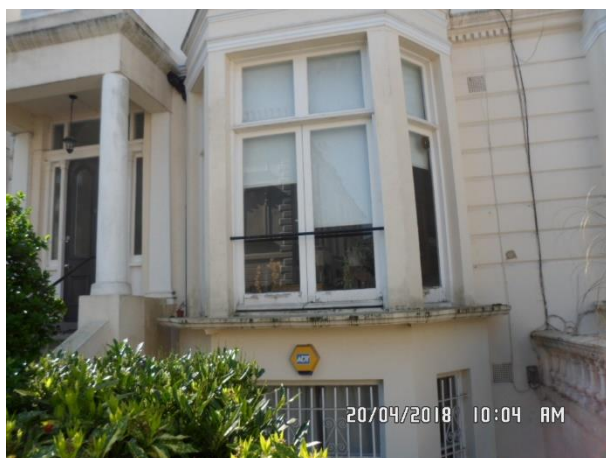
18 Belsize Square Front Elevation to Building
