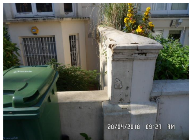
18 Belsize Square Front to Front Boundary Wall
