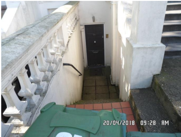
18 Belsize Square Front Elevation Steps Down to Flat
