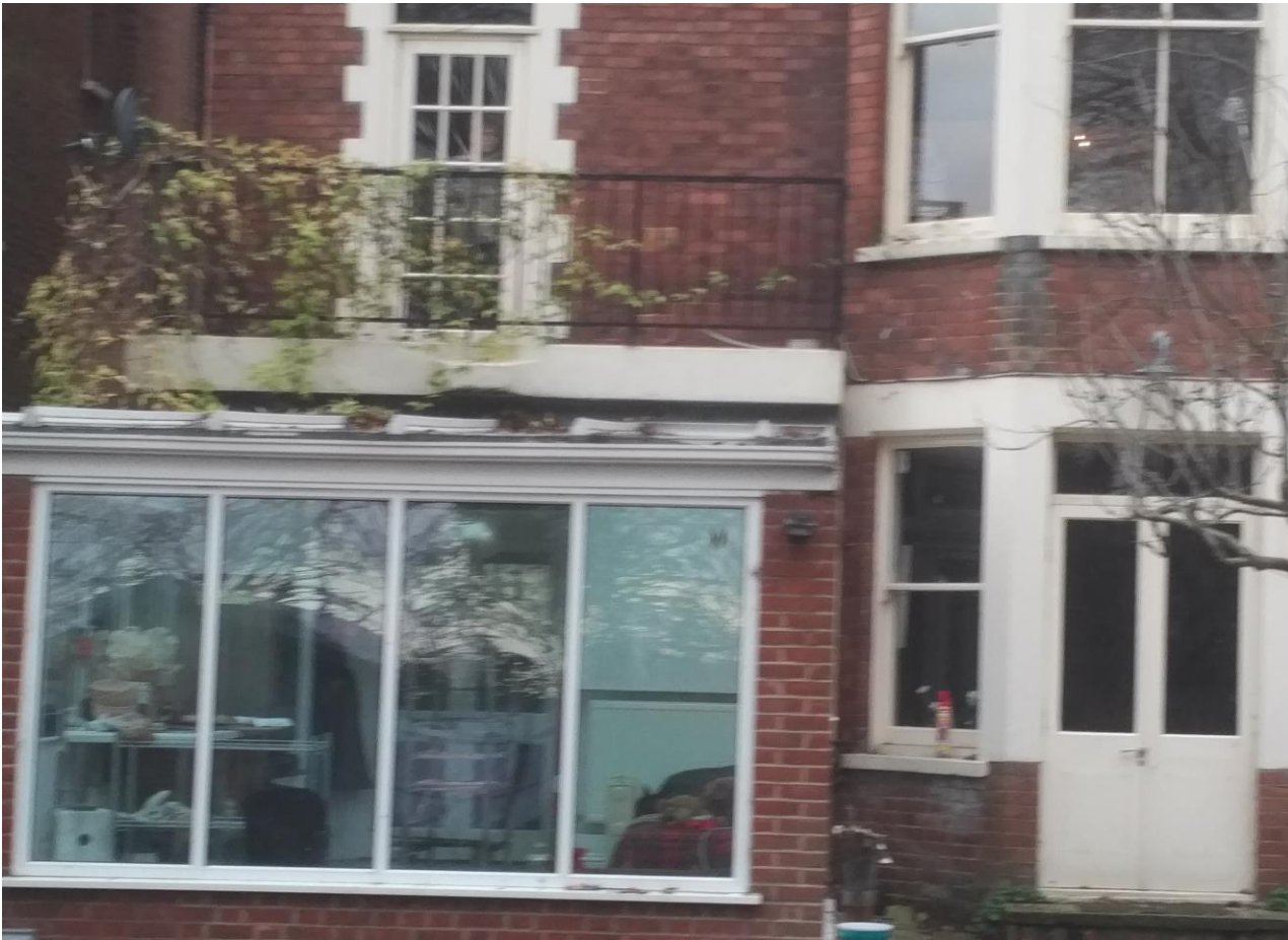
Example of larger rear extension and terrace (No.25)
