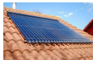
Figure 6 – Solar Thermal Panels
