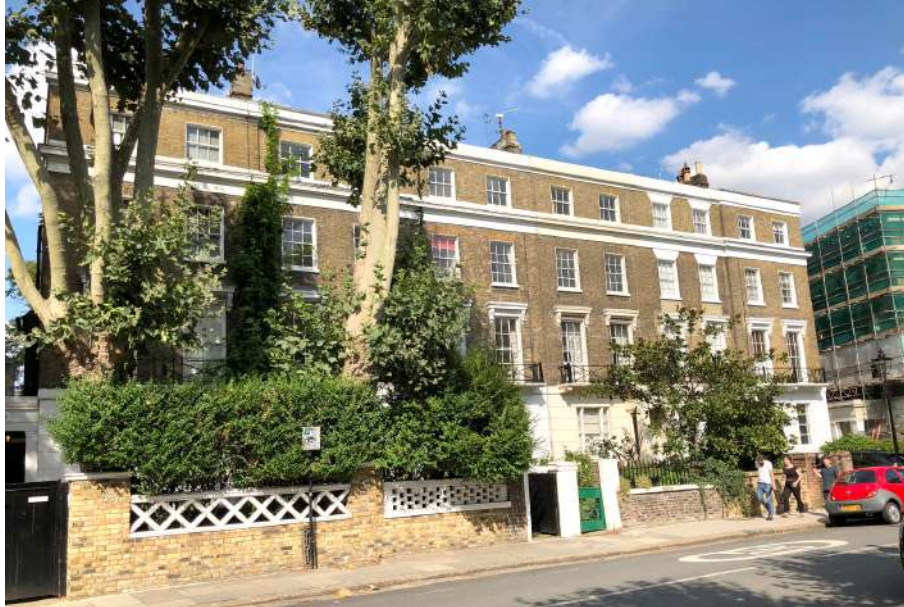
Fig 2 Street View of No. 35 to 30 Gloucester Crescent
