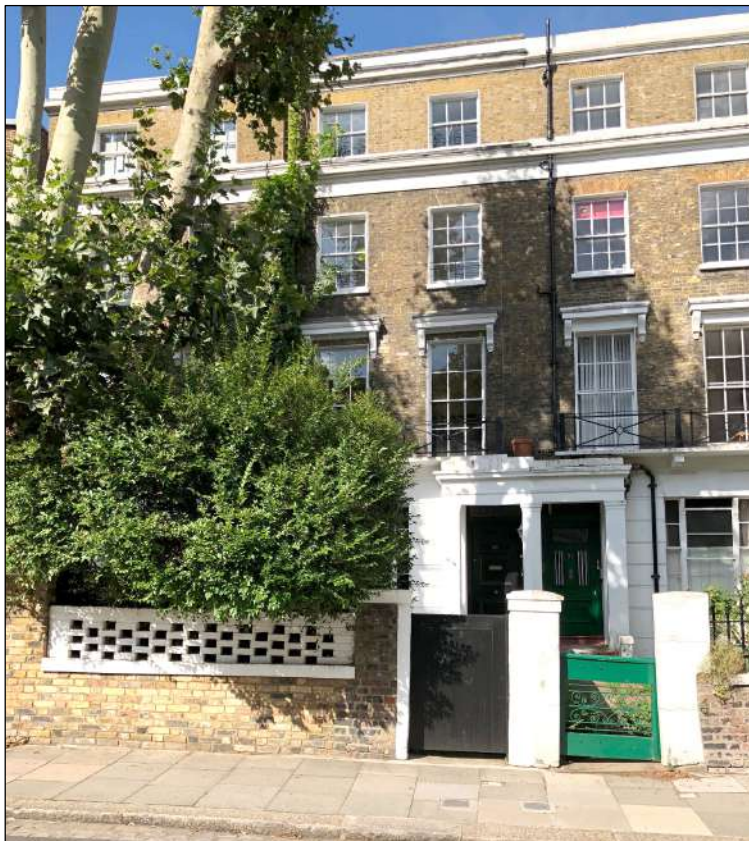
Fig 3 Front View of No. 34 Gloucester Crescent.
