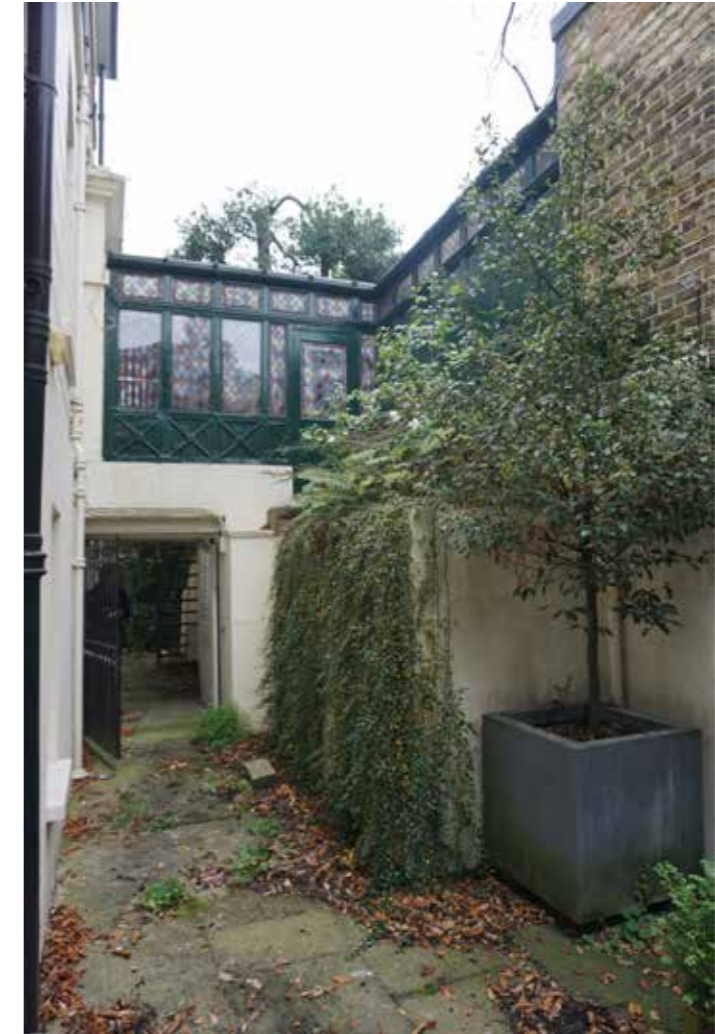
Existing planter structure
