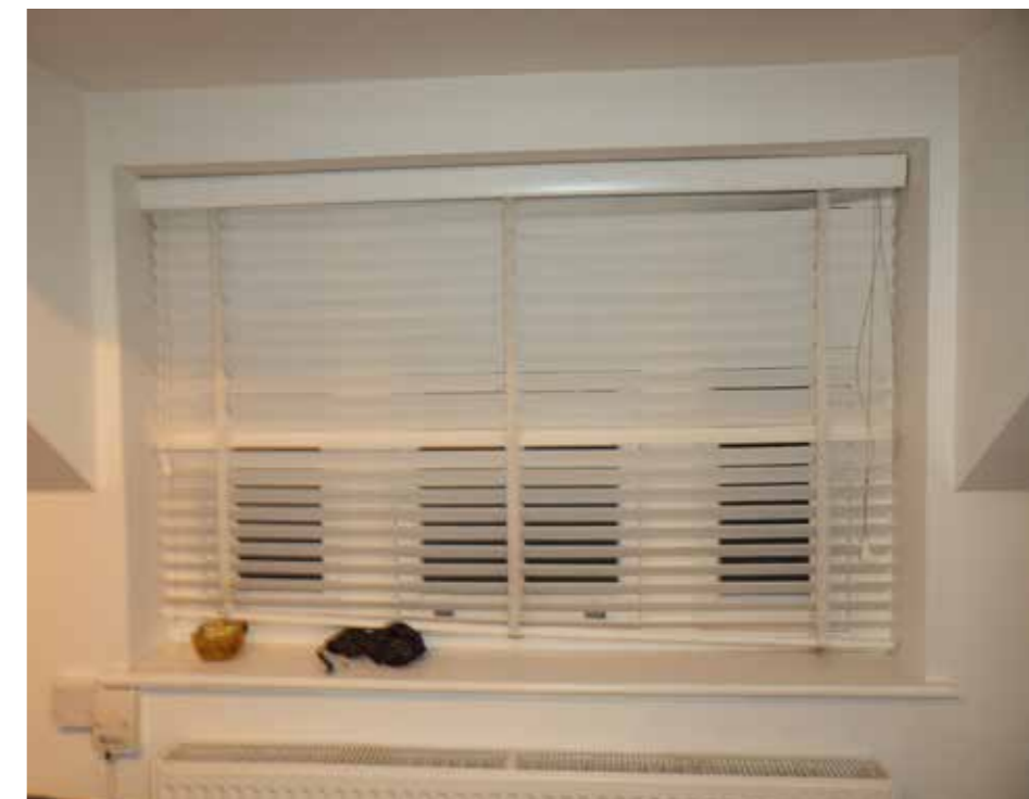
Existing window WGF-11
