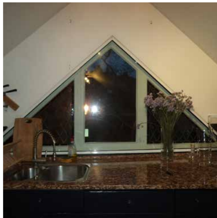
Existing window WGF-12
