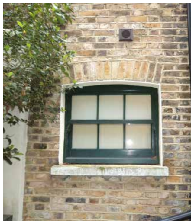
External view of existing window WLGF-10
