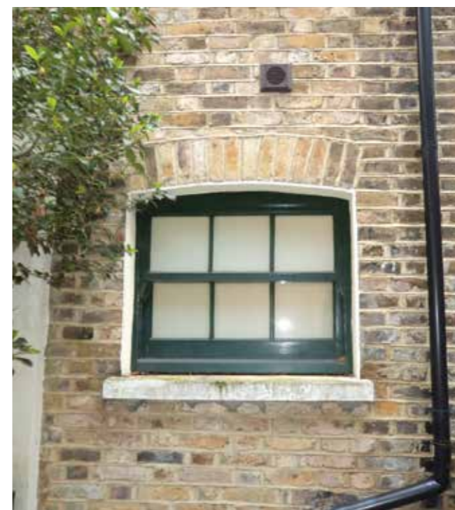
Repairs to brickwork
