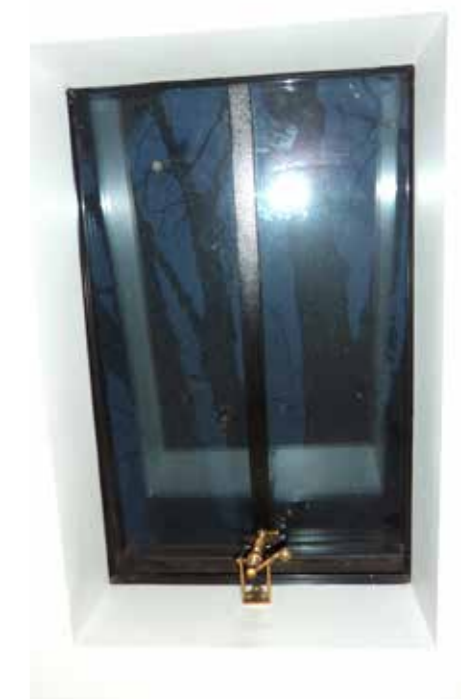
Existing roof light WRL-02
