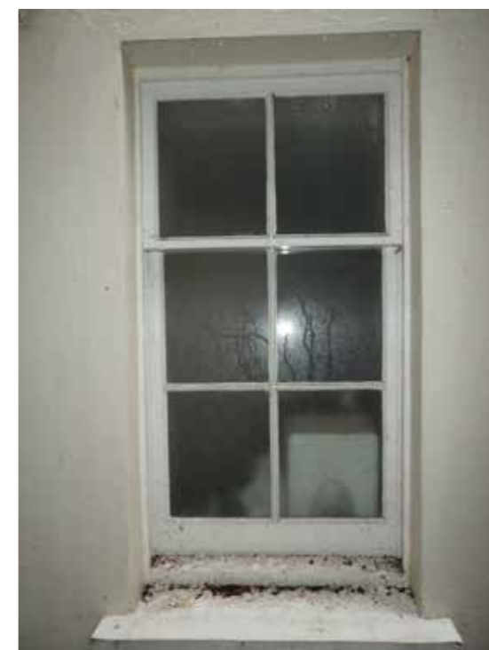
External view of existing window WLGF-09
