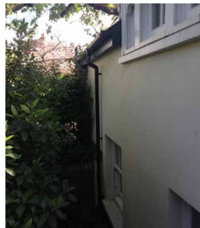
Repairs to gutters
