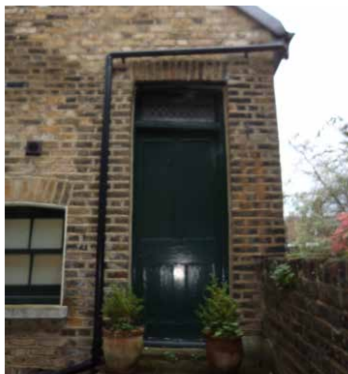
Repairs/rationalising rainwater goods
