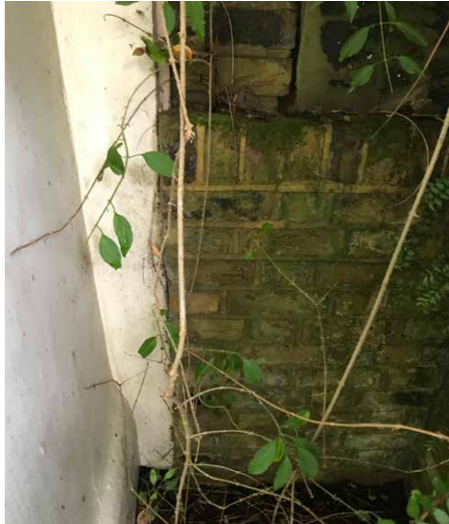
Existing area of brick boundary wall
