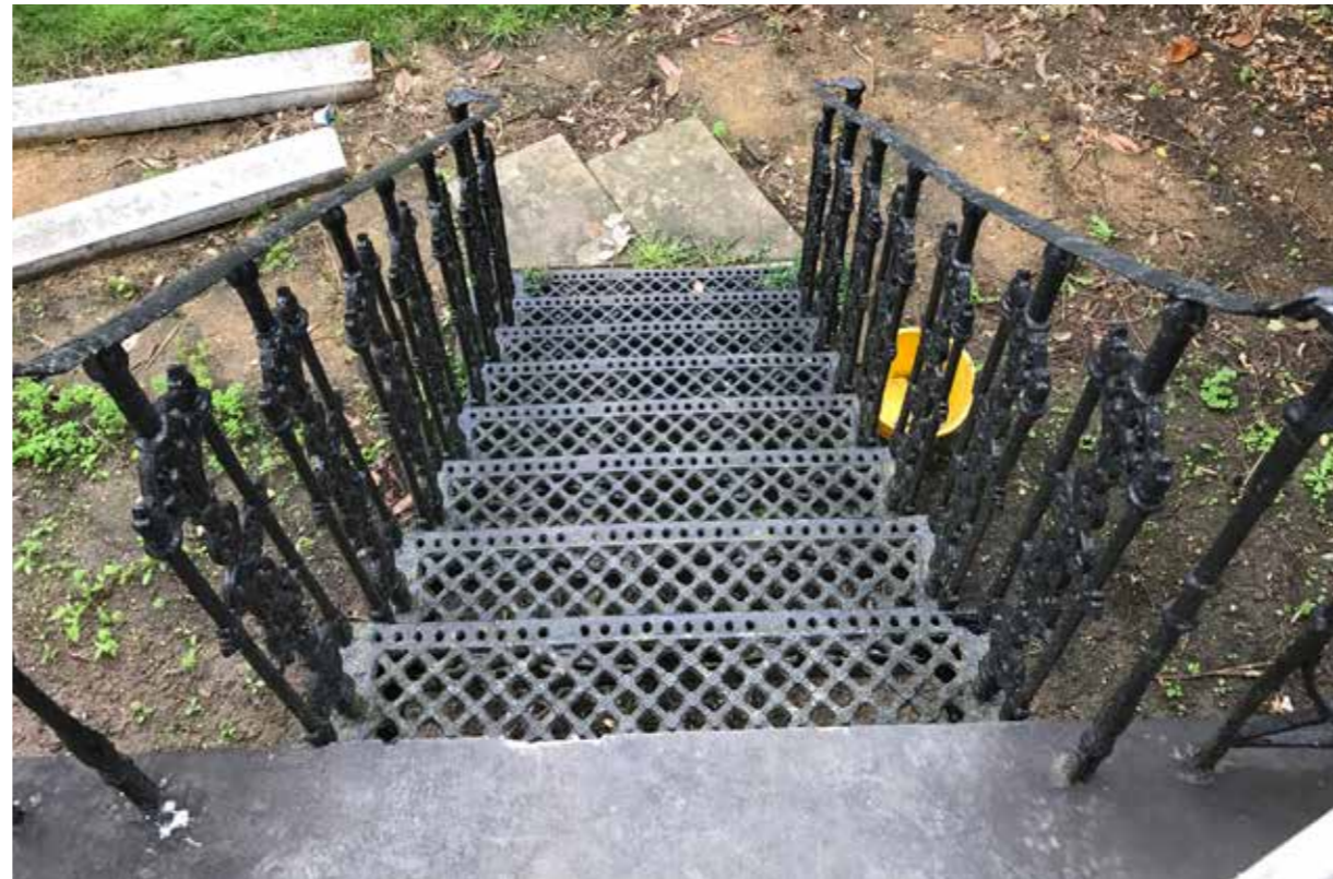
Existing GF balcony staircase
