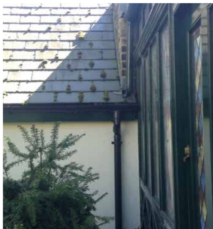
Repairs/rationalising rainwater goods
