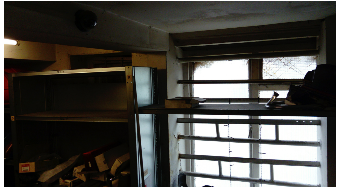
EXISTING WINDOW LOOKING OUT TOWARDS THE REAR COURTYARD AT THE BACK
