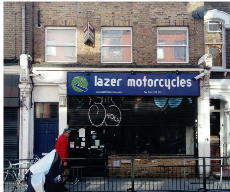
PHOTO OF EXISTING FRONTAGE
