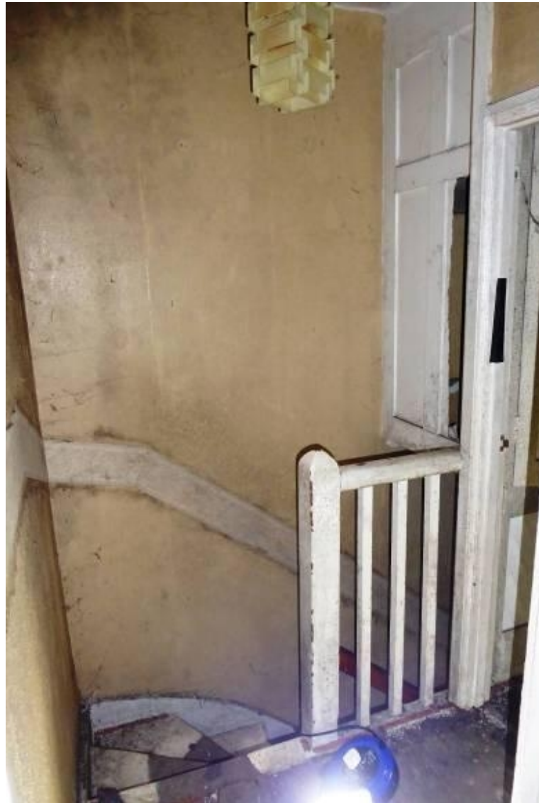
Fig 5.3.11: Landing with balustrade at door to front bedroom
