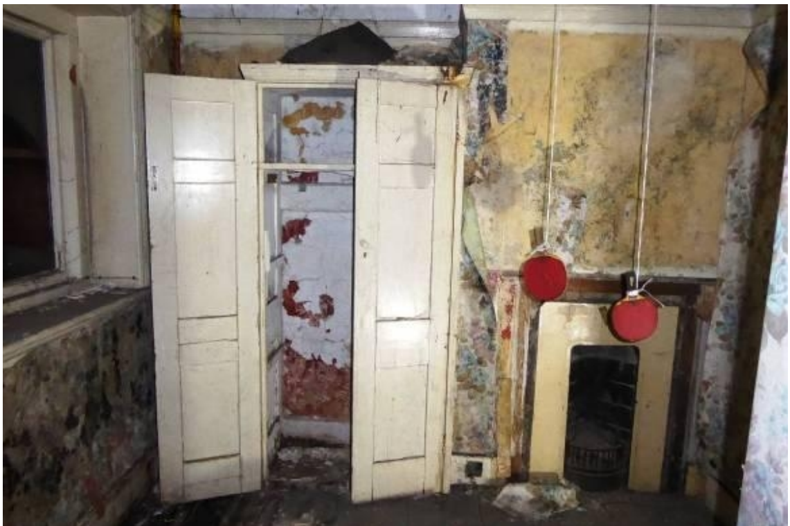
Fig 5.2.14: Rea bedroom cupboard
