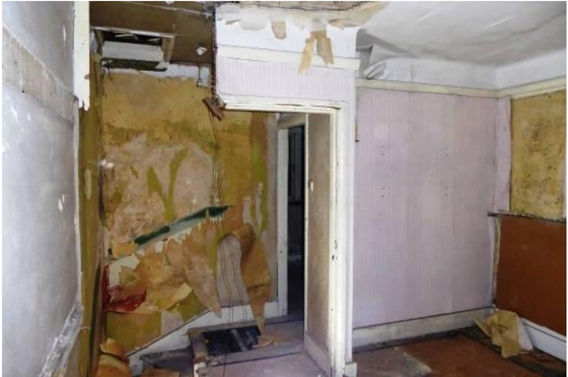
Fig 4.7: Landing from front bedroom through removed wall
