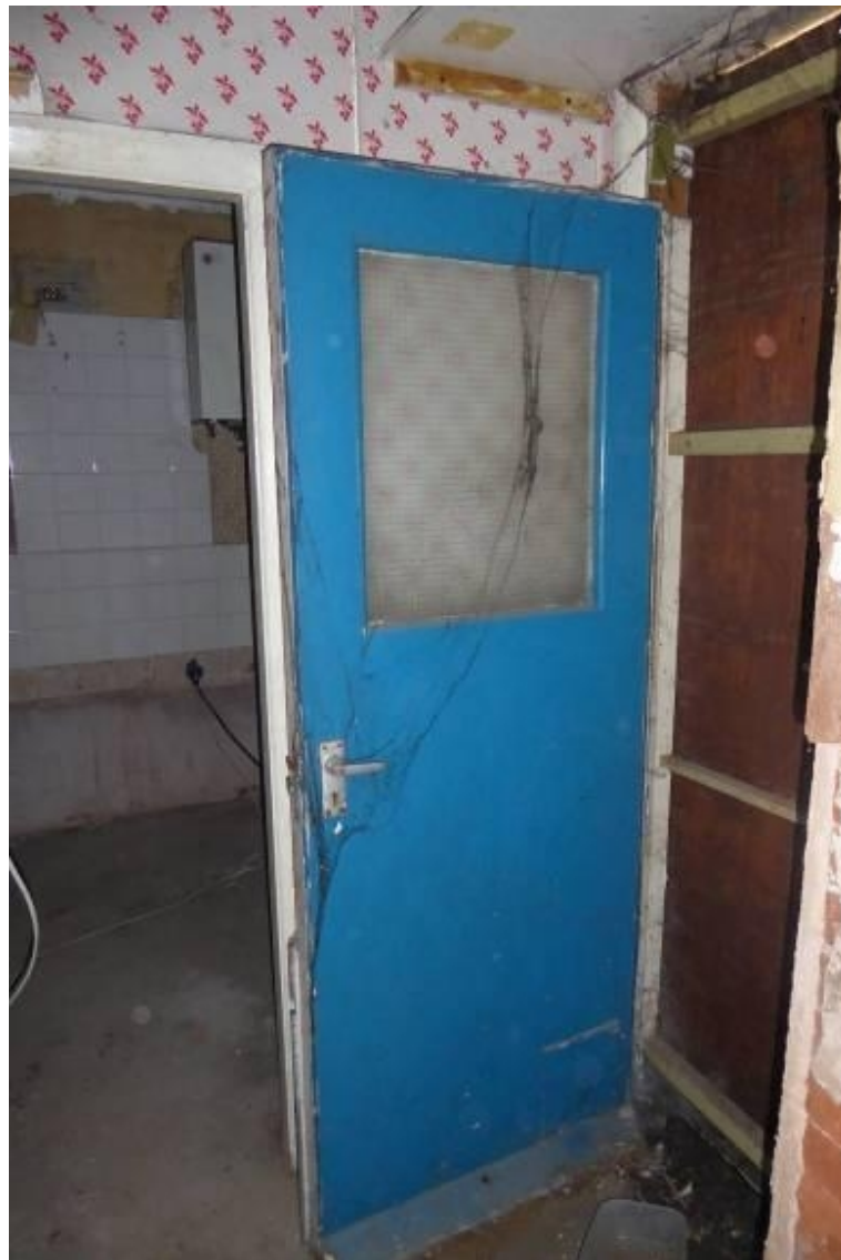
Fig 4.4: Bathroom / rear entrance lobby with external door
