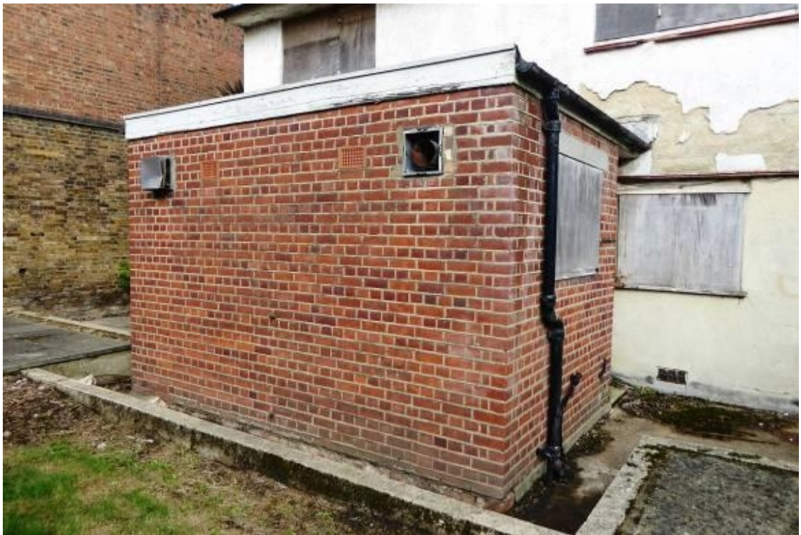
Fig 3.5.12: Rear extension walls
