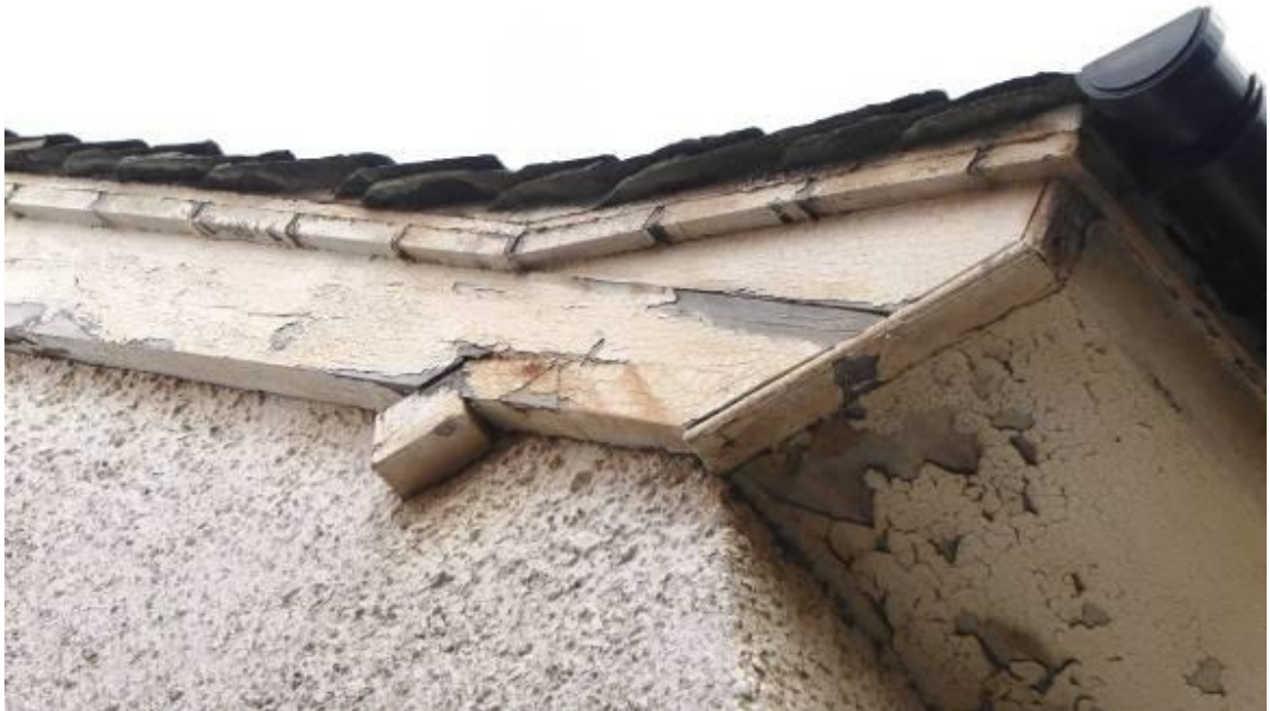
Fig 3.3.1: Main roof eaves and gable junction
