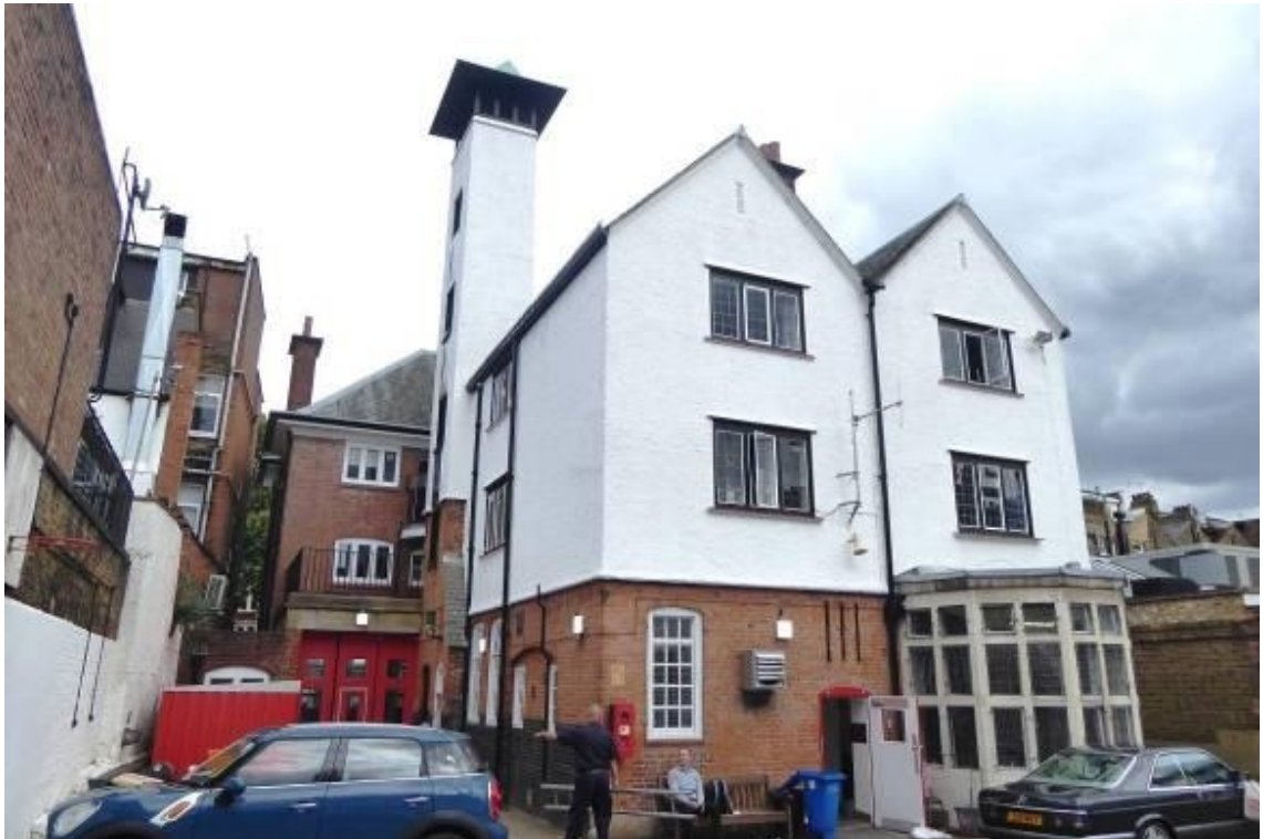
Fig 2.1.2: West End Lane Fire Station rear
