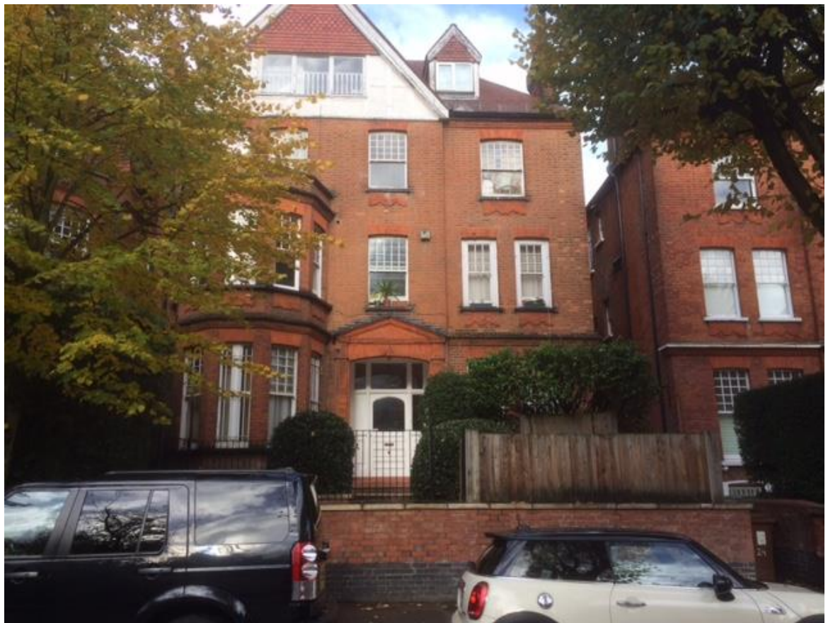
Photograph 2: Front Elevation of 24 Wedderburn Road
