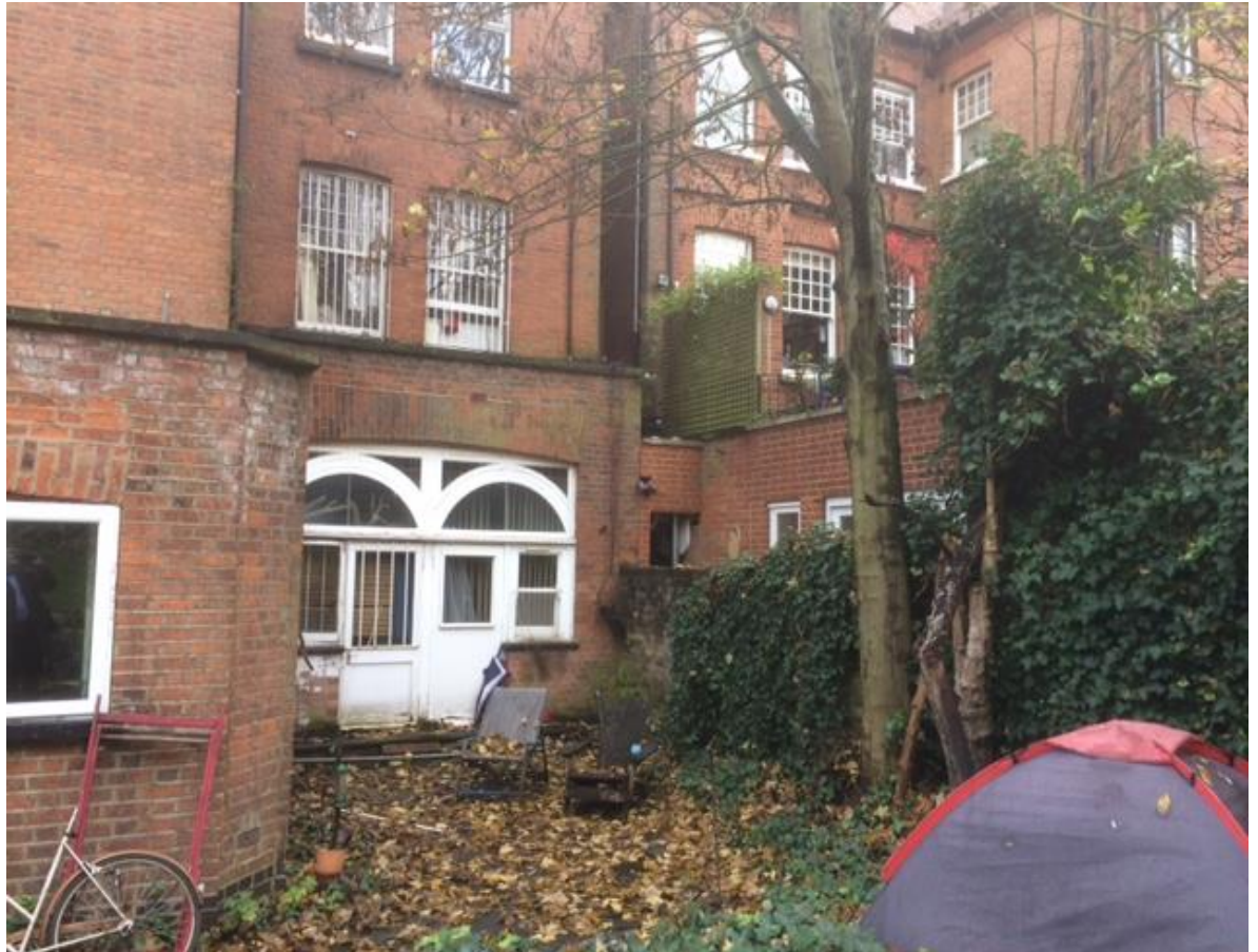
Photograph 3: Back Elevation of 24 Wedderburn Road
