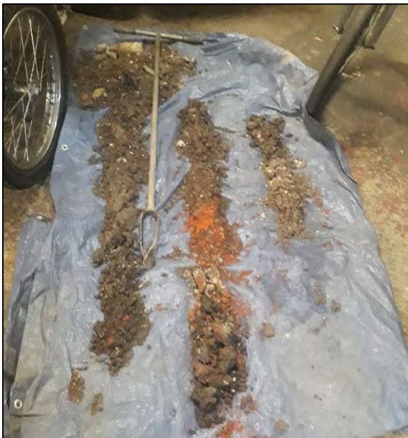
Image 2: Excavations at BH01.
