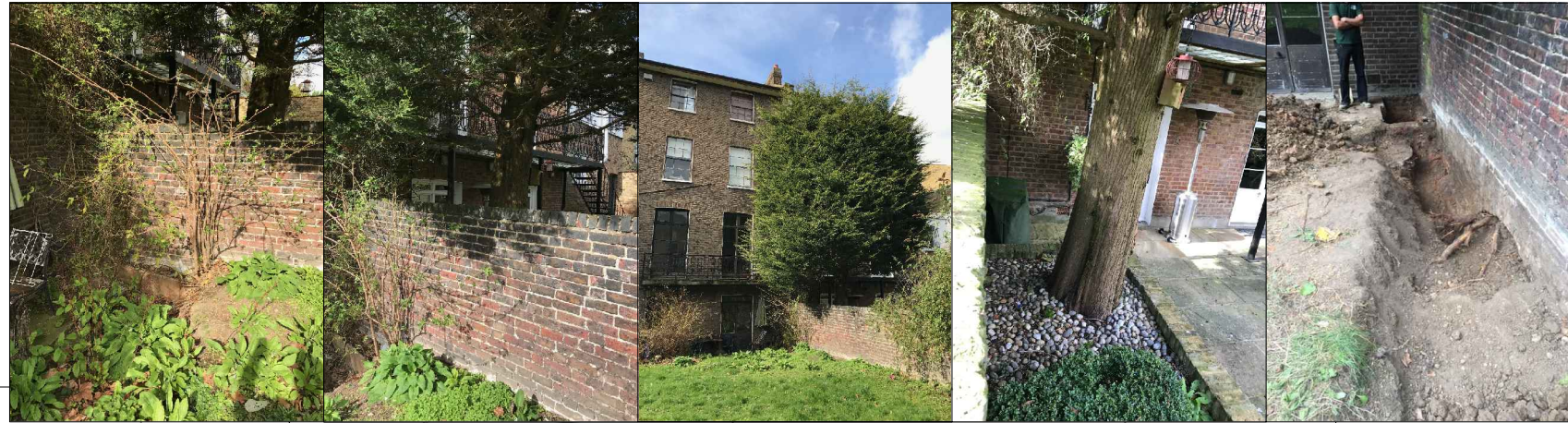
Tree root investigation along boundary to inform RPA of T3.
