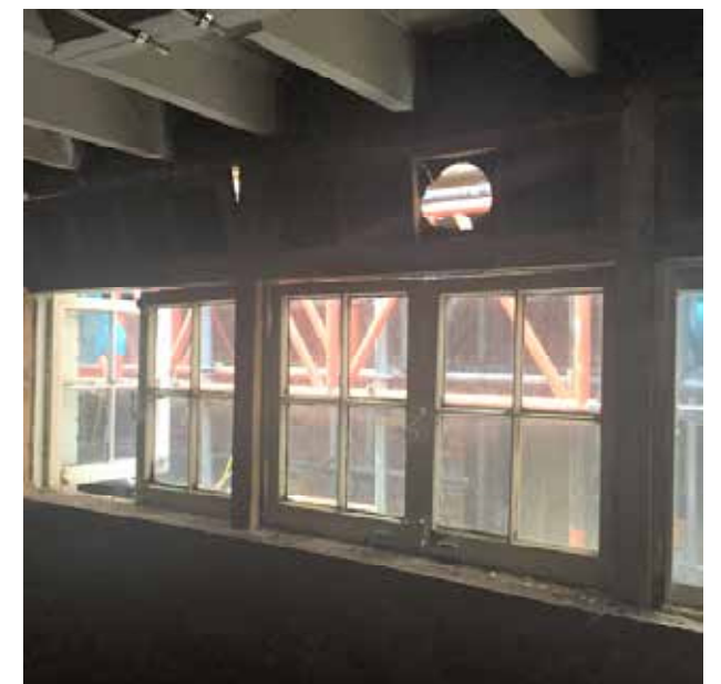
First Floor casement windows with later lining and lipping removed to reveal fanlights and window frames
