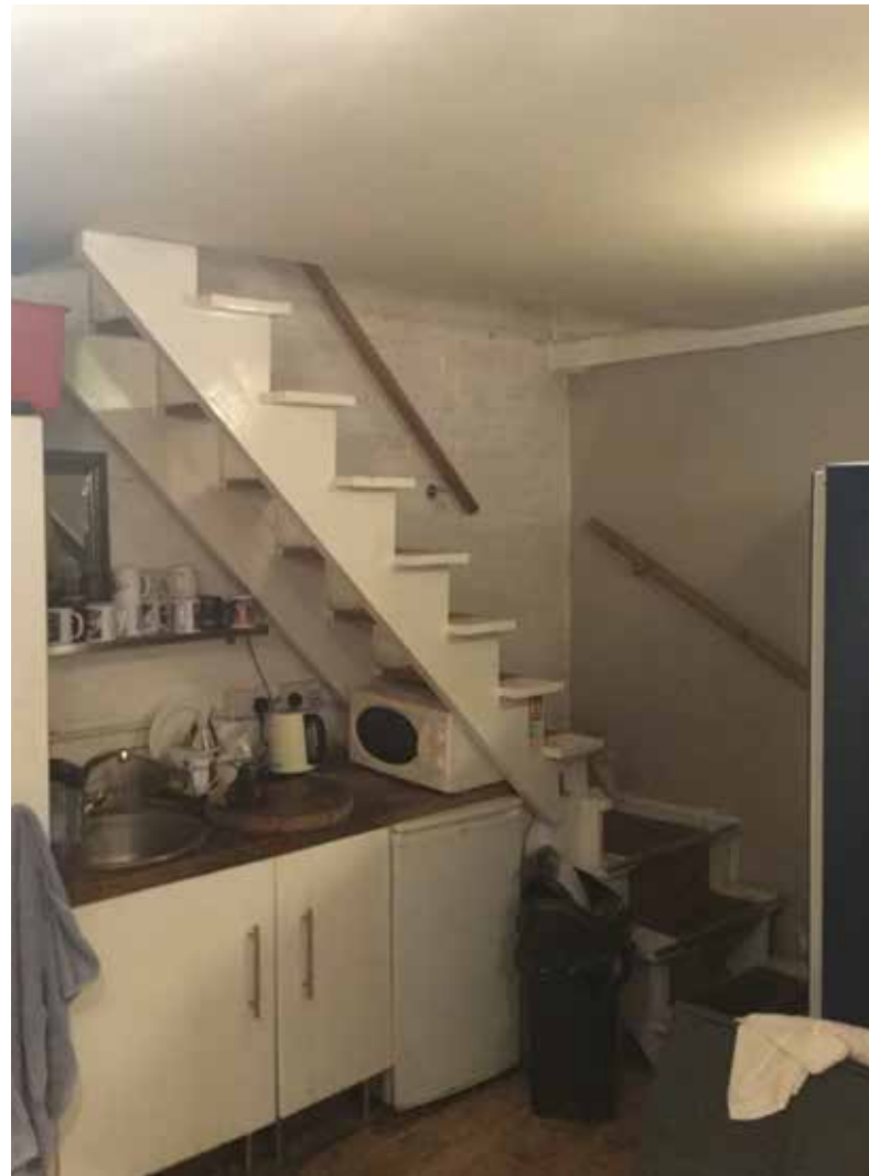
Temporary staircase to be removed, cupboard and kitchen units below stairs have been stripped out as agreed with Historic England.
