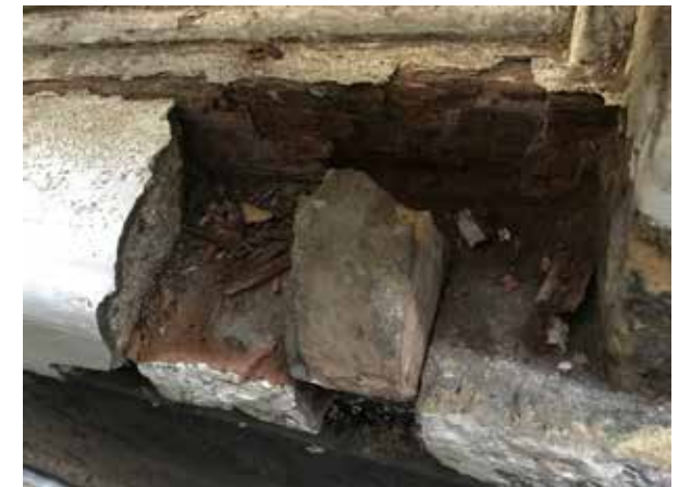
Photo of rotten external cill, ground floor
