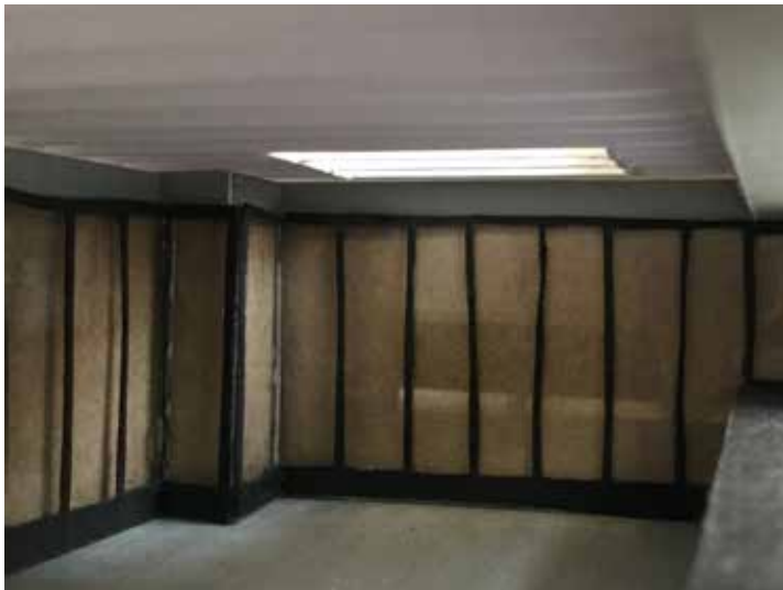
Option 2 Full height glazing with expressed frame between joints. This option exposes the full length of artwork but the framing could detract from the artwork,
