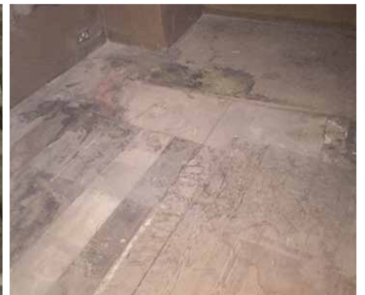
Areas of ply boarding covering original floor boards
