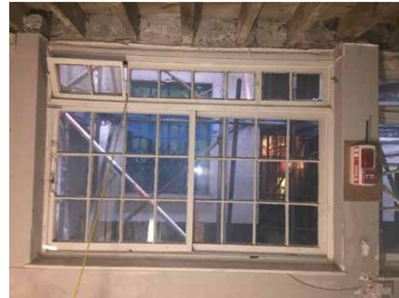
Photo of ground floor Yorkshire sliding windows, ground floor
